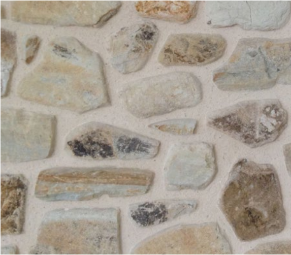
Natural rocks set in mortar / concrete in areas of high water flow
