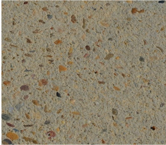
Exposed aggregate concrete paving Non-slip finish
