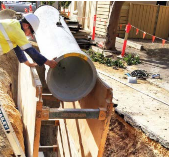
Stormwater infrastructure upgrades
