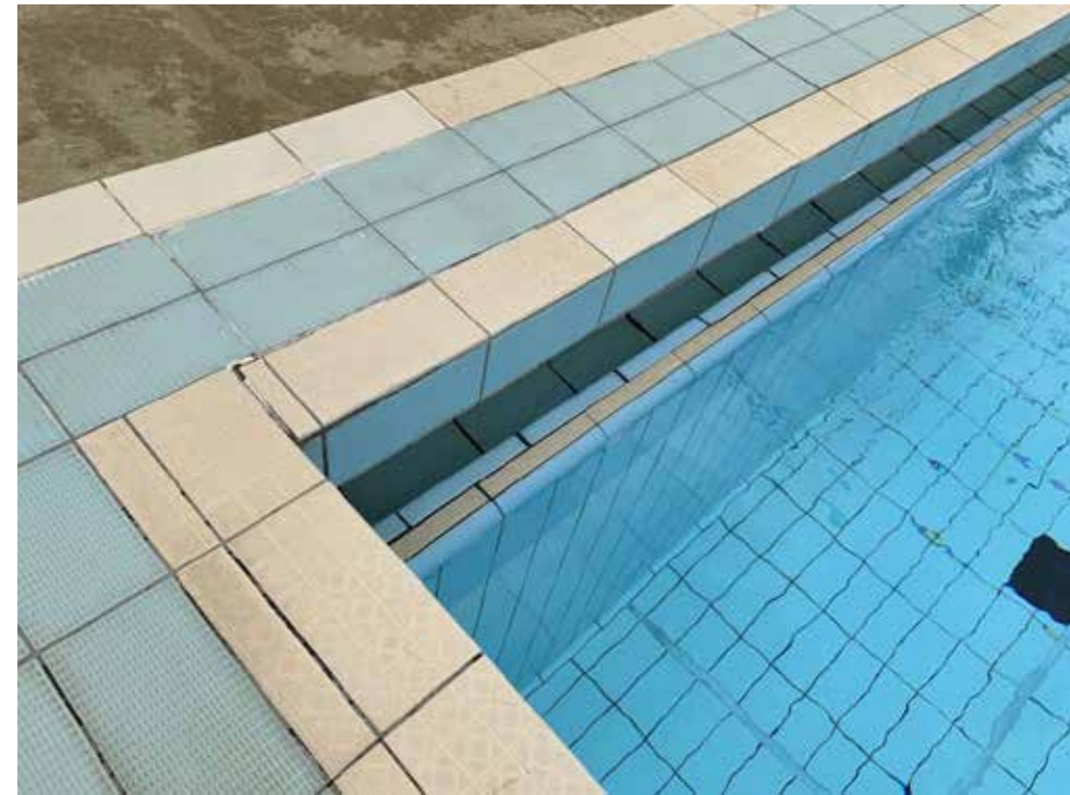
Figure 6: 50m Scum Gutter Removal system
