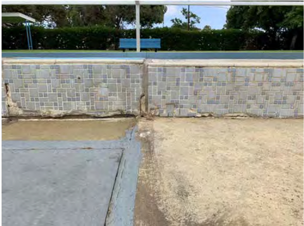
Figure 12: Movement in pool structure at central joint
