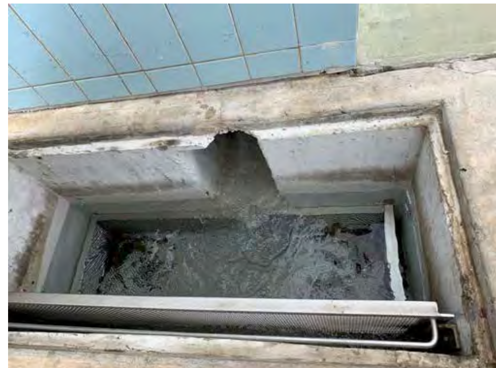
Figure 7: Scum gutter outlets at ends of channel
