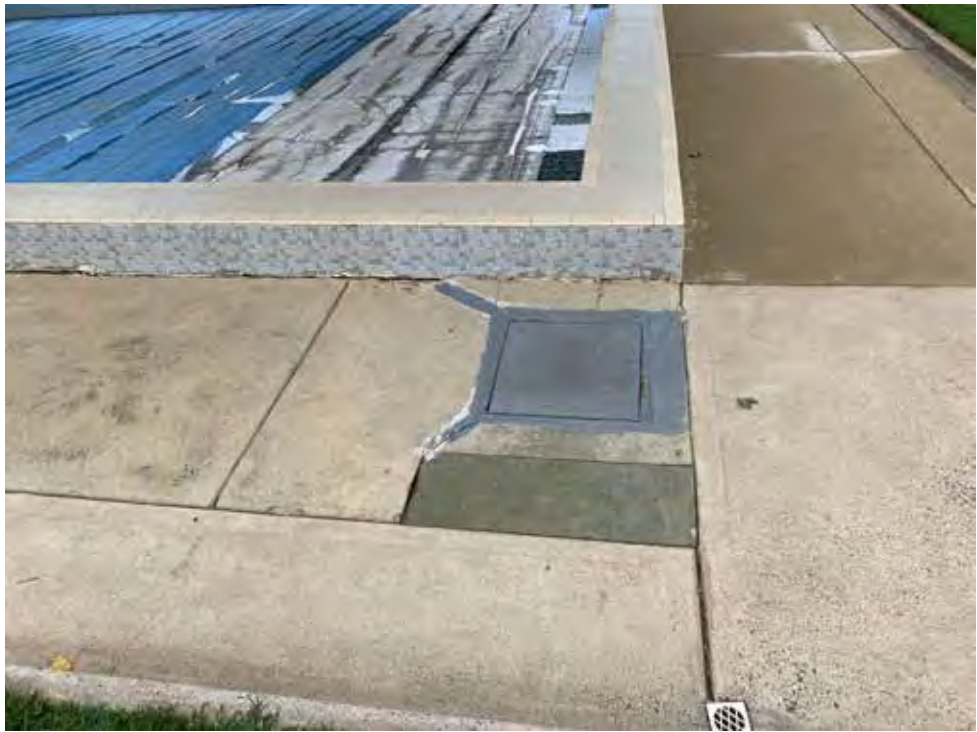
Figure 13: Concourse subsidence in corner of pool
