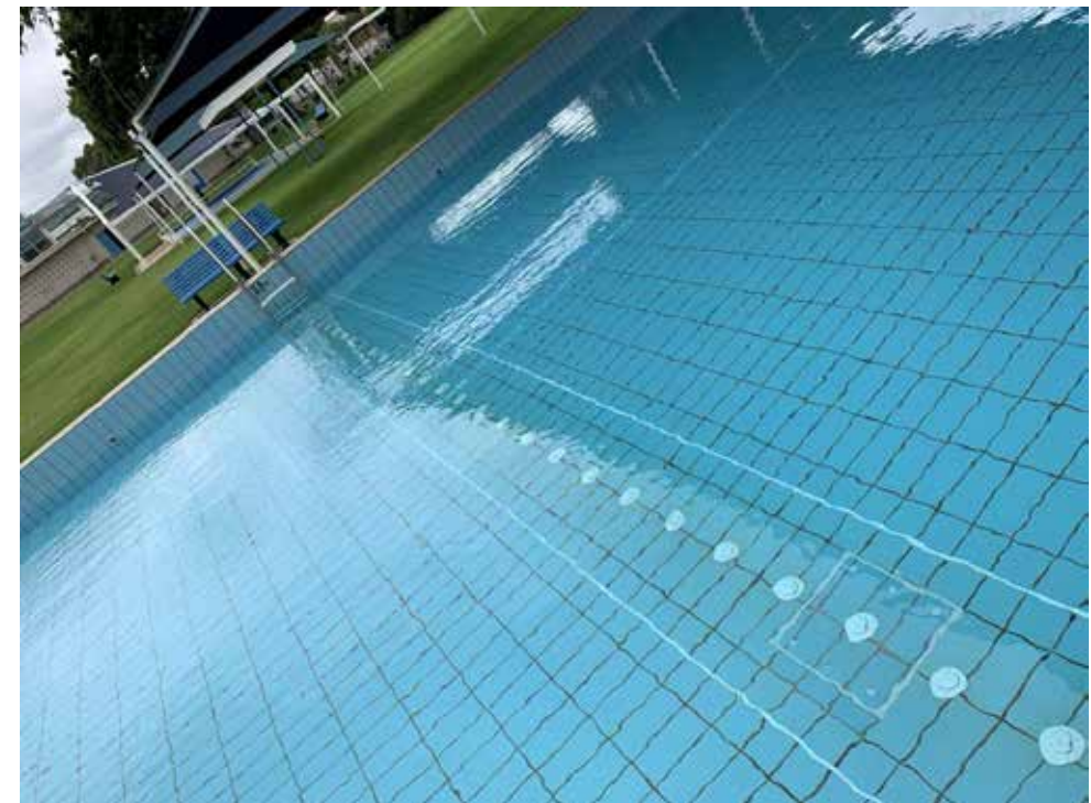
Figure 10: Floor returns in pool
