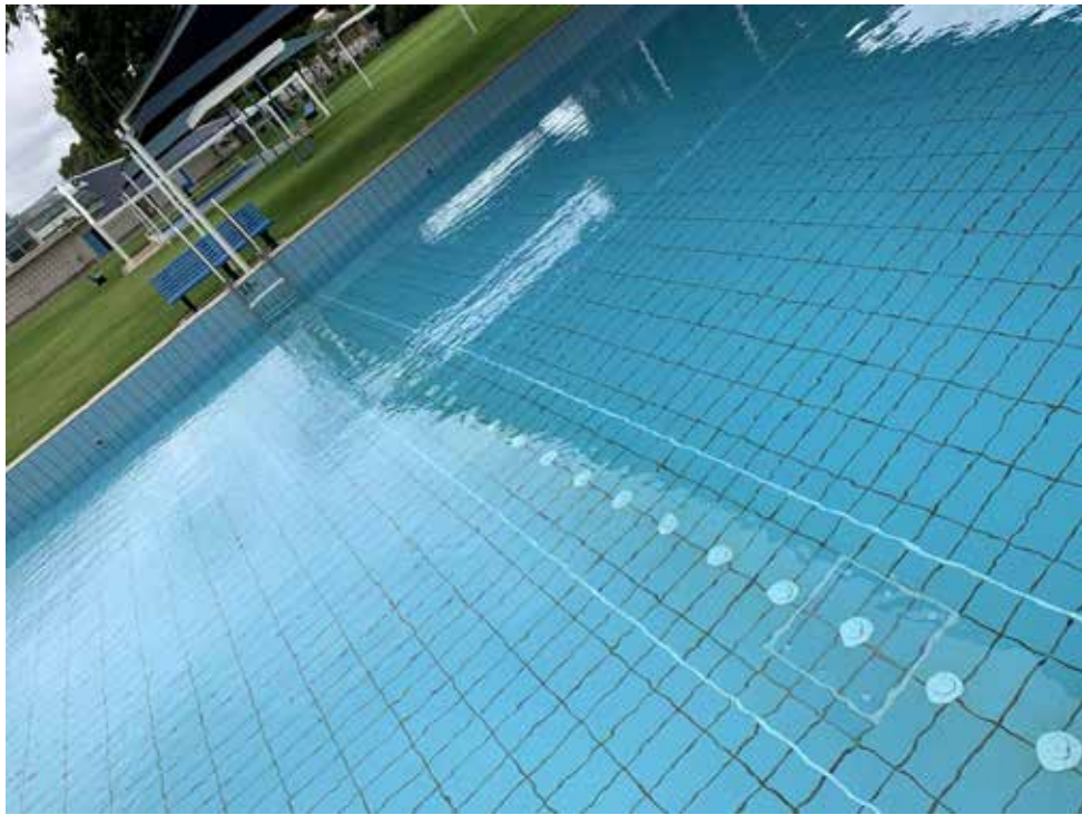
Figure 10: Floor returns in pool
