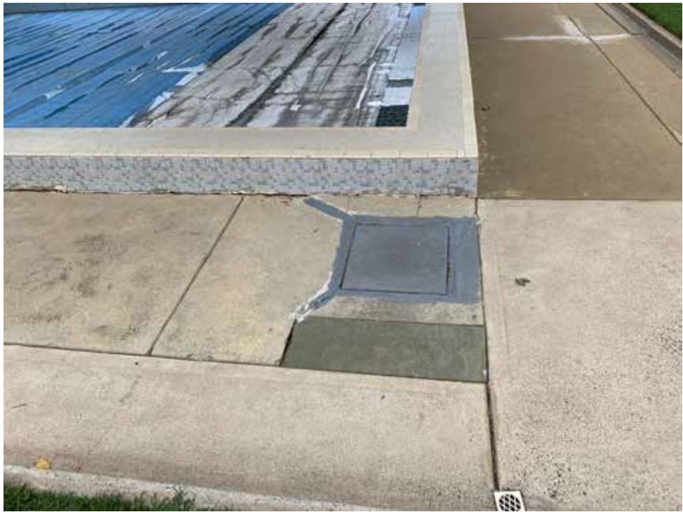
Figure 13: Concourse subsidence in corner of pool
