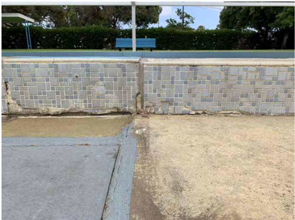
Figure 12: Movement in pool structure at central joint
