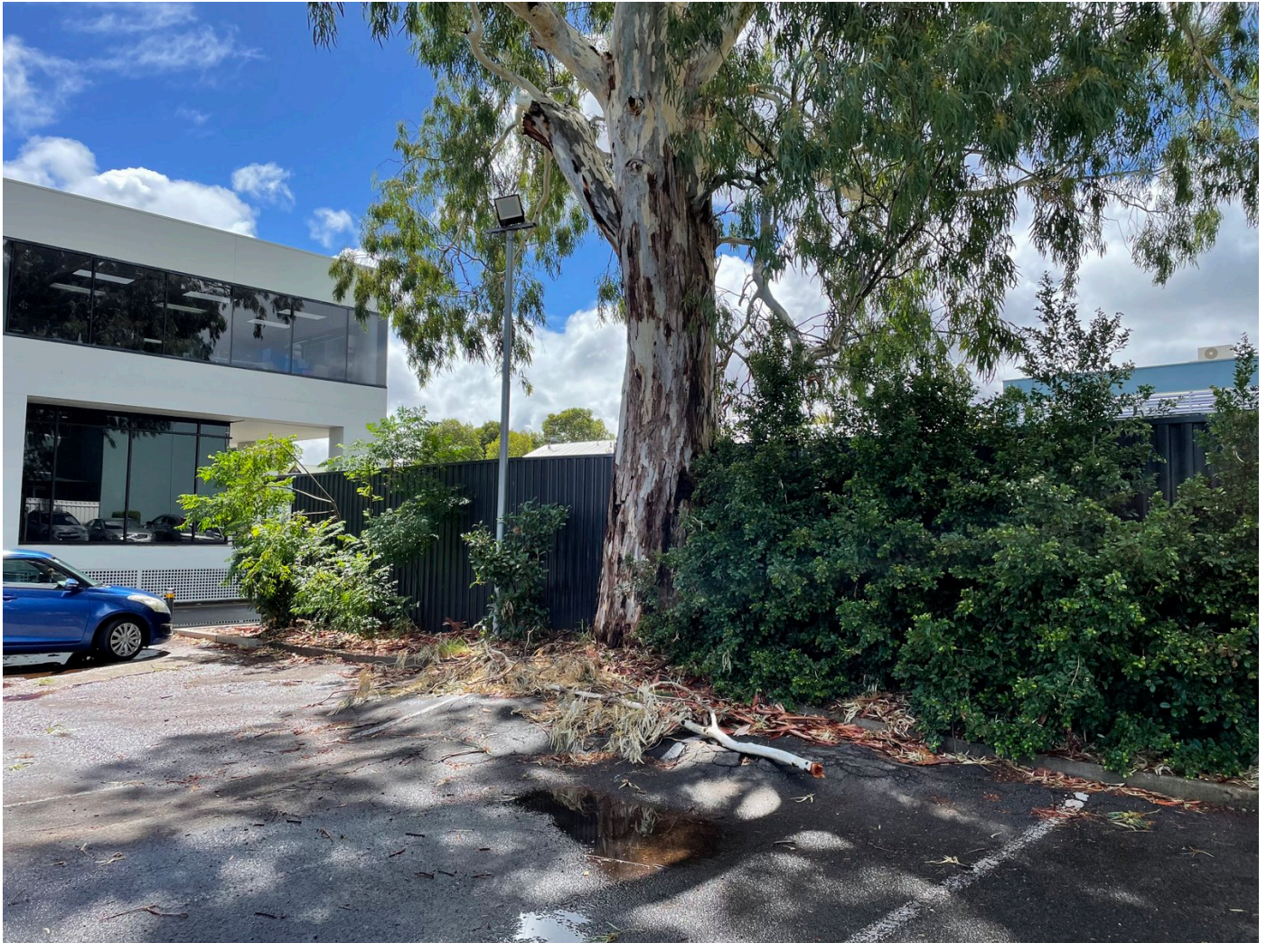
Figure 17. My photograph of the subject tree, looking approximately north-east from the Britannia Hotel carpark on the 8 th of March 2023. There is up to 500 mm of vertical displacement of the bitumen-sealed surface of both the carpark at the Britannia Hotel carpark and the carpark in the allotment of 37-39 Wadham Lane, caused by an ongoing increase in the diameter of the roots of the tree. The concrete edge to the carpark at the Britannia Hotel has also been displaced by the tree.
