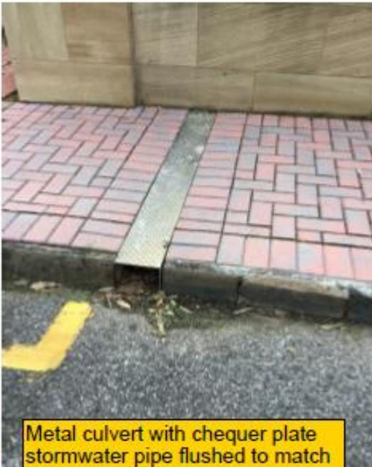
Metal culvert with chequer plate stormwater pipe flushed to match footpath levels
