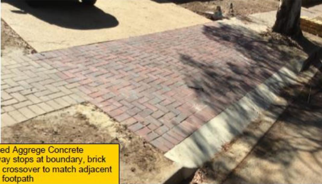
Exposed Aggregate Concrete driveway stops at boundary, brick paved crossover to match adjacent paved footpath
