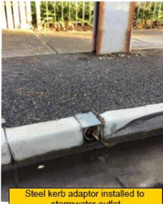
Steel kerb adaptor installed to stormwater outlet
