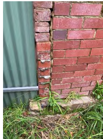
Figure 22: Rear paths required to control water pooling against the building's edge.
