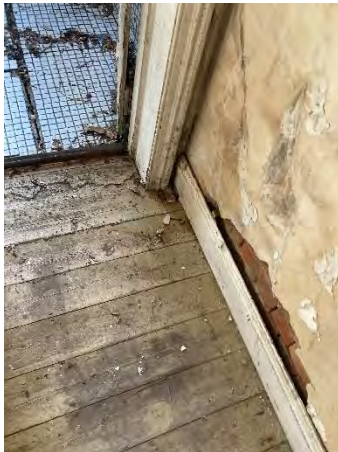
Figure 53: Damp walls require a chemical treatment, once dried out.
