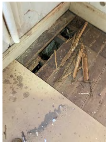
Figure 61: Past termite damage to floor joists, boards and skirting, require treatment and repair.
