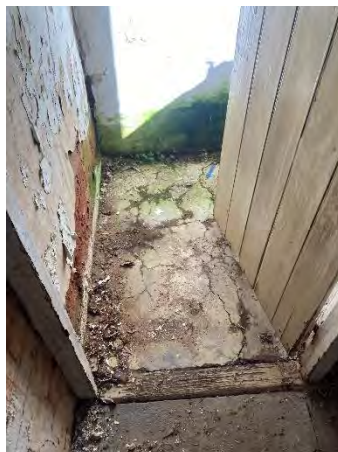
Figure 69: Internal doors and door frames require repair or replacement.
