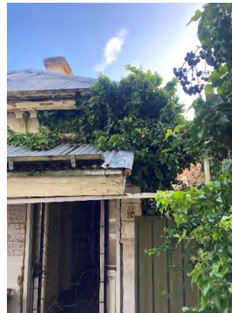
Figure 3: Replace front verandah, posts, supports, fascia, sheeting, gutters and downpipes.
