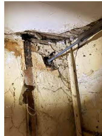
Figure 52: Extensive removal of and repairs and / or replacement of solid render required.
