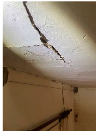
Figure 43: Extensive repairs and / or new ceilings required to dwelling.
