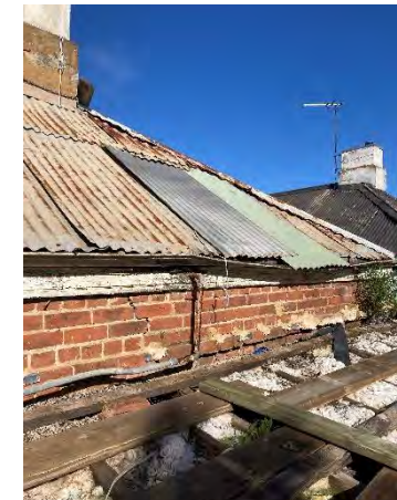
Figure 27: New roof sheeting , gutter and flashing is required.
