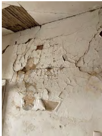
Figure 54: Damp walls require a chemical treatment, once dried out.
