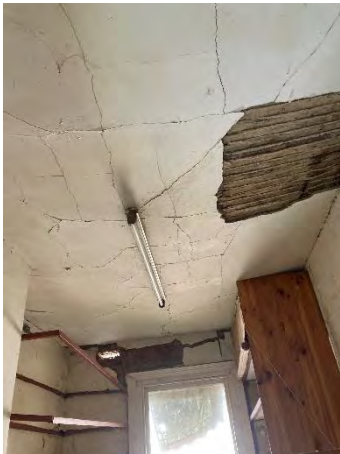
Figure 41: Extensive repairs and / or new ceilings required to dwelling.
