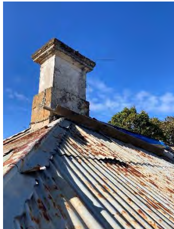
Figure 33: Chimney repairs required.
