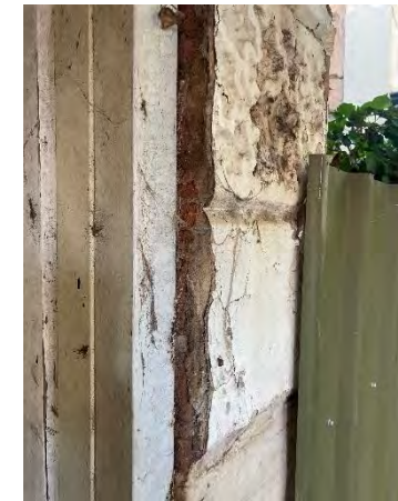
Figure 8: Repairs to brick work, salt damp, quoin work required to front facade.
