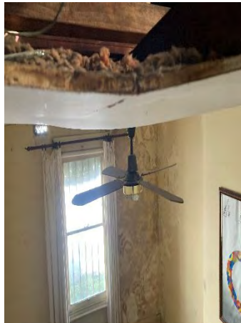
Figure 59: Damp walls require a chemical treatment, once dried out.
