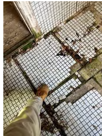
Figure 78: Loose pavement squares to bathroom floor.
