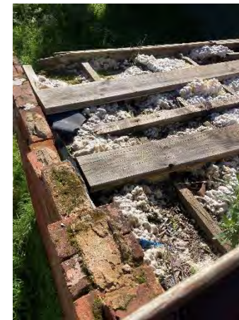
Figure 95: Roof framing requires upgrading and additional support.
