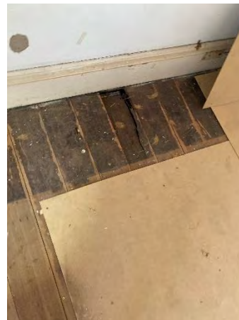
Figure 62: Past termite damage to floor joists, boards and skirting, require treatment and repair.
