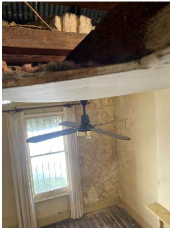
Figure 92: Roof framing requires upgrading and additional support.
