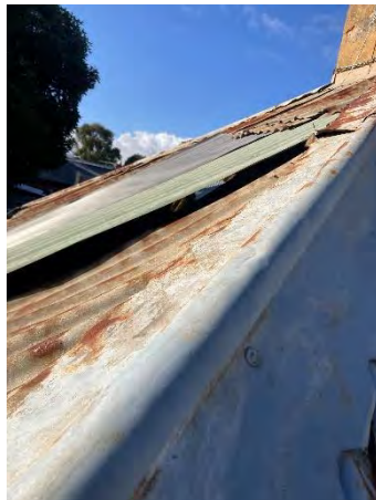
Figure 24: New roof sheeting , gutter and flashing is required.
