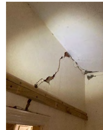
Figure 48: Extensive removal of and repairs and / or replacement of solid render required.
