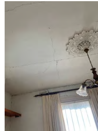
Figure 39: Extensive repairs and / or new ceilings required to dwelling.
