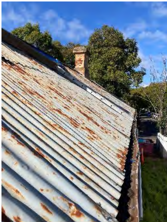
Figure 23: New roof sheeting , gutter and flashing is required.
