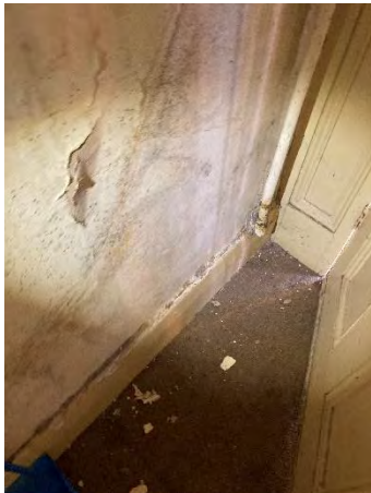
Figure 58: Damp walls require a chemical treatment, once dried out.
