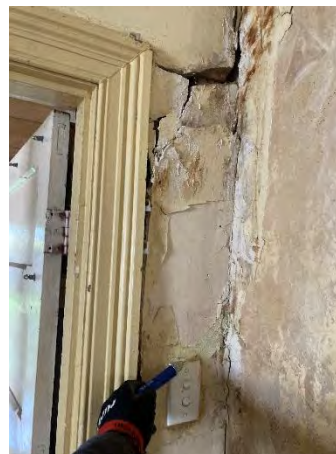
Figure 66: Wiring requires upgrading and safety repairs.
