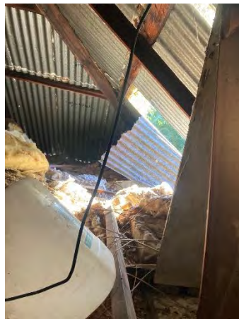
Figure 93: Roof framing requires upgrading and additional support.
