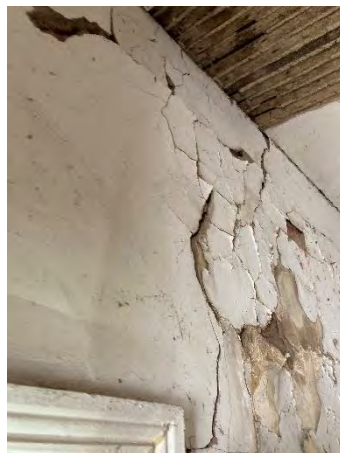
Figure 45: Extensive removal of and repairs and / or replacement of solid render required.
