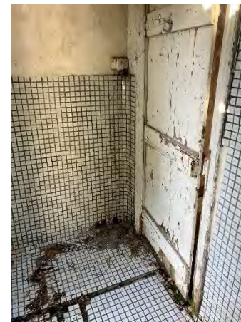
Figure 71: Internal doors and door frames require repair or replacement.
