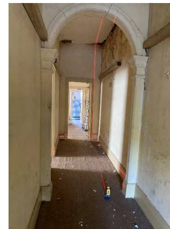
Figure 47: Extensive removal of and repairs and / or replacement of solid render required.
