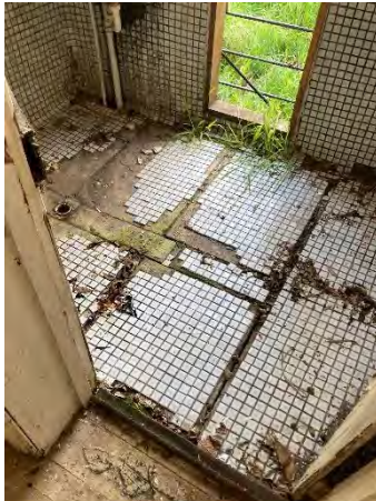
Figure 76: New bathroom fit out required, including waterproofing, tiles, sanitaryware. No allowance made for new sewer line.
