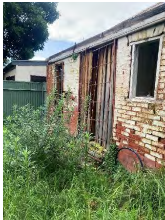
Figure 21: Rear paths required to control water pooling against the building's edge.
