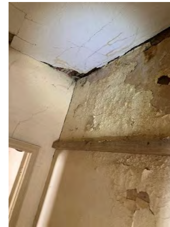
Figure 56: Damp walls require a chemical treatment, once dried out.
