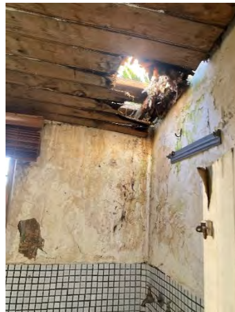
Figure 77: New bathroom fit out required, including waterproofing, tiles, sanitaryware. No allowance made for new sewer line.
