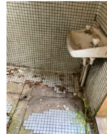
Figure 80: New bathroom fit out required, including waterproofing, tiles, sanitaryware. No allowance made for new sewer line.
