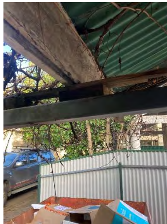
Figure 2: Replace front verandah, posts, supports, fascia, sheeting, gutters and downpipes.
