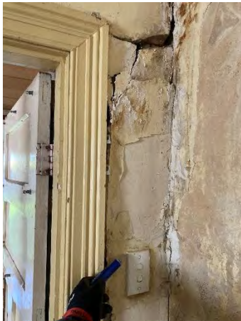
Figure 49: Extensive removal of and repairs and / or replacement of solid render required.
