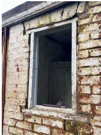
Figure 29: New windows and doors to the rear required. Repairs required to the western side and front façade.
