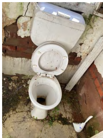
Figure 90: WC walls, ceiling and sanitaryware require replacement.
