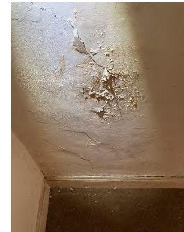
Figure 57: Damp walls require a chemical treatment, once dried out.
