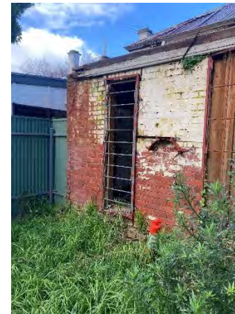
Figure 31: New windows and doors to the rear required. Repairs required to the western side and front façade.
