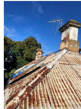
Figure 26: New roof sheeting , gutter and flashing is required.
