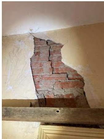
Figure 50: Extensive removal of and repairs and / or replacement of solid render required.
