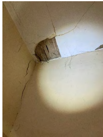
Figure 37: Extensive repairs and / or new ceilings required to dwelling.
