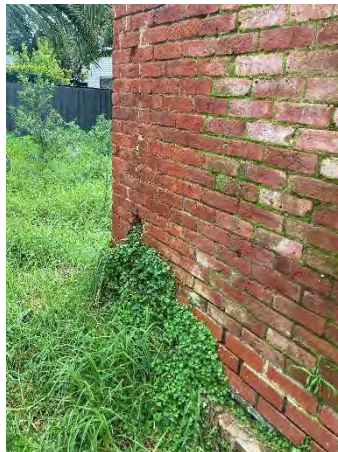
Figure 14: Install base and driveway to control water pooling against the building's edge.
