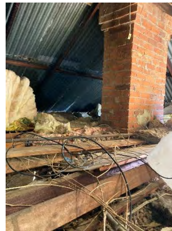
Figure 94: Roof framing requires upgrading and additional support.
