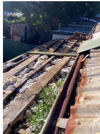
Figure 25: New roof sheeting , gutter and flashing is required.
