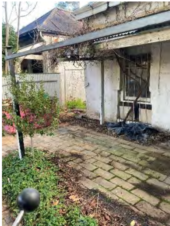
Figure 1: Replace front verandah, posts, supports, fascia, sheeting, gutters and downpipes.
