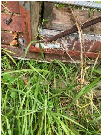
Figure 20: Rear paths required to control water pooling against the building's edge.
