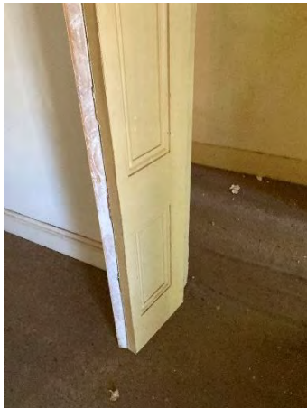
Figure 68: Internal doors and door frames require repair or replacement.
