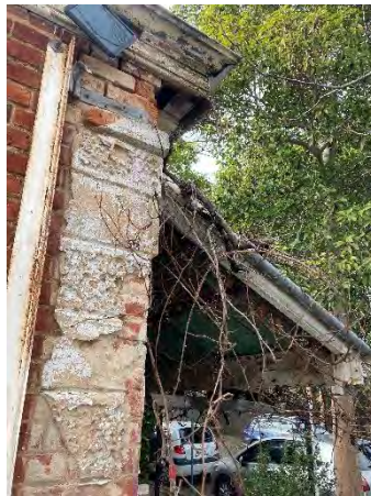
Figure 5: Repairs to brick work, salt damp, quoin work required to front facade.
