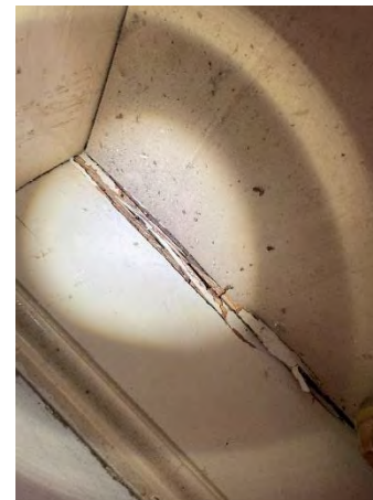
Figure 63: Past termite damage to floor joists, boards and skirting, require treatment and repair.
