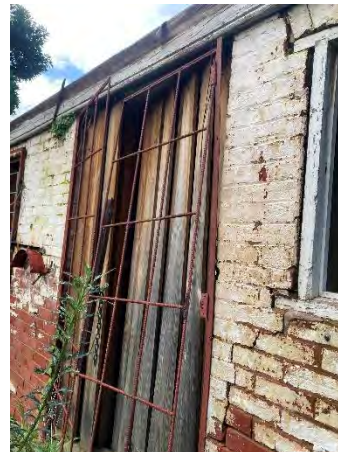
Figure 30: New windows and doors to the rear required. Repairs required to the western side and front façade.
