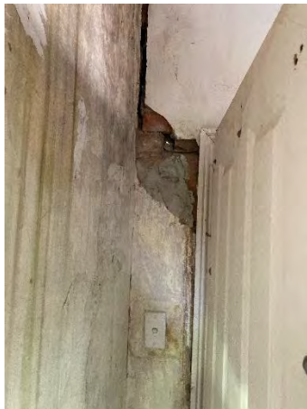
Figure 44: Extensive removal of and repairs and / or replacement of solid render required.
