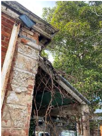
Figure 97: External and internal painting required.
