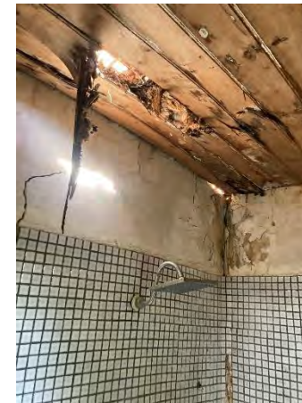
Figure 79: New bathroom fit out required, including waterproofing, tiles, sanitaryware. No allowance made for new sewer line.
