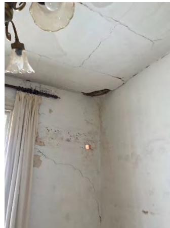
Figure 55: Damp walls require a chemical treatment, once dried out.
