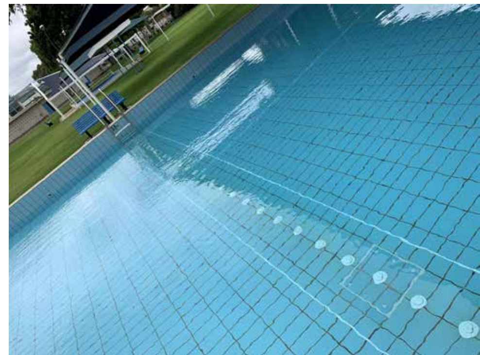
Figure 10: Floor returns in pool
