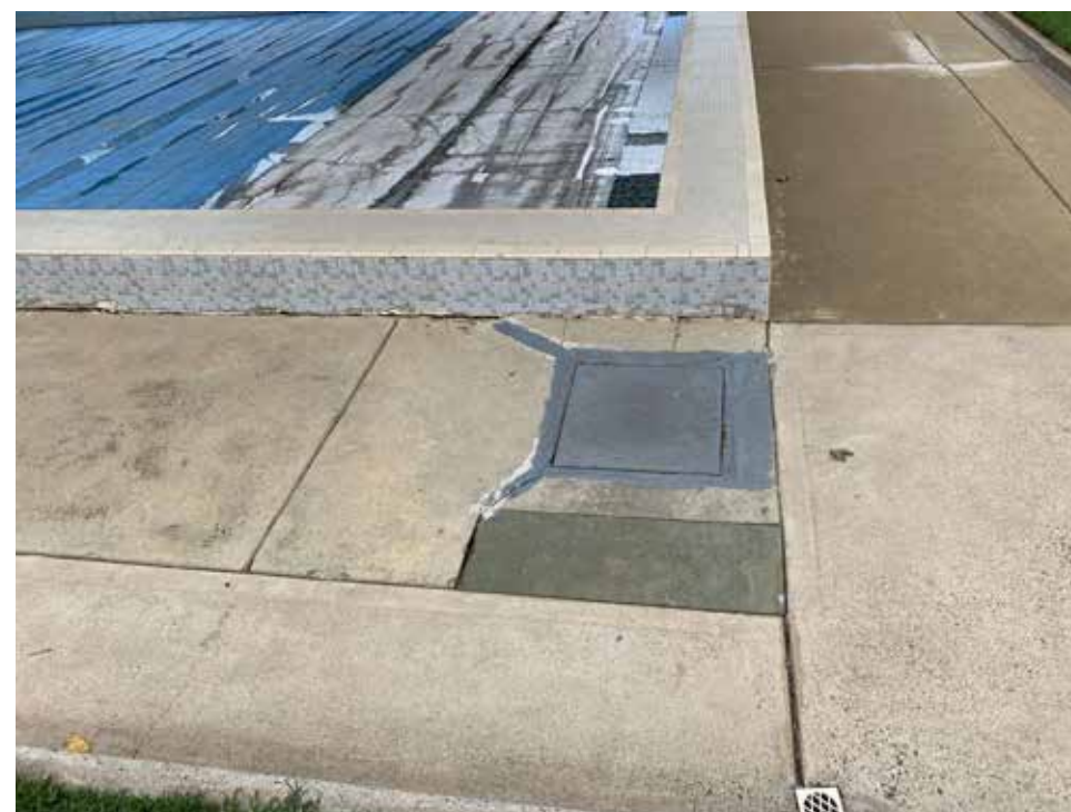
Figure 13: Concourse subsidence in corner of pool
