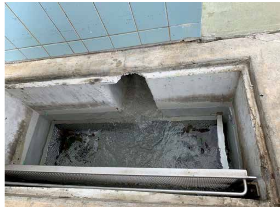
Figure 7: Scum gutter outlets at ends of channel
