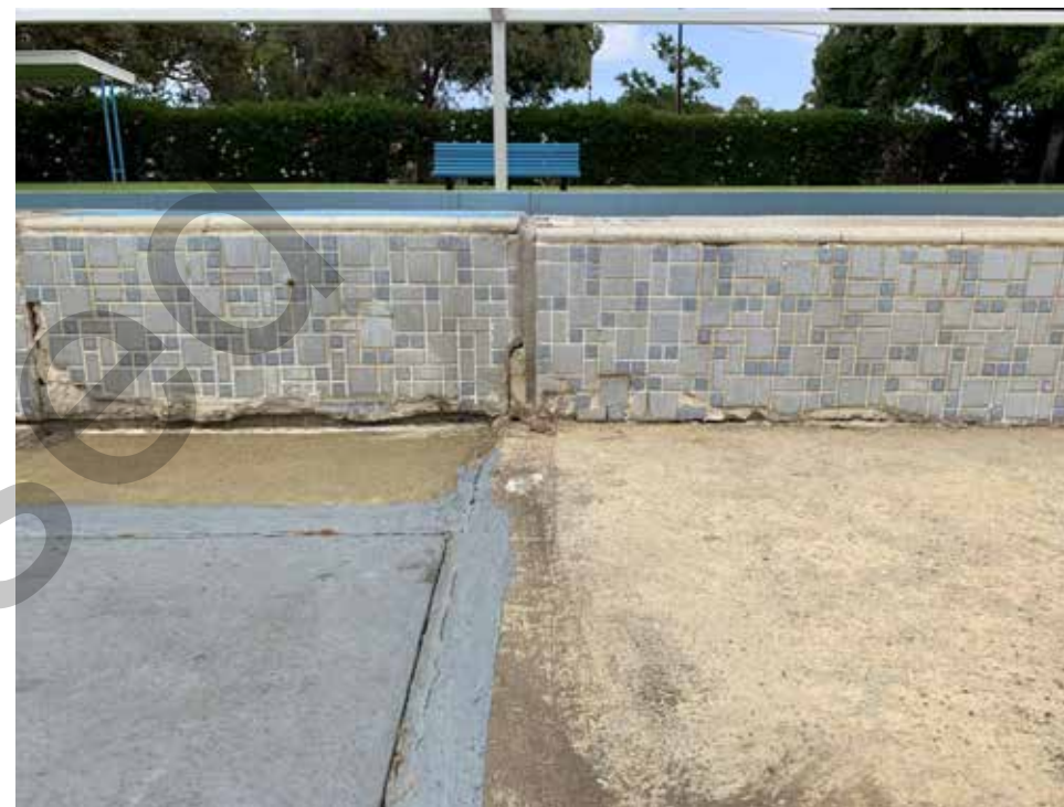
Figure 12: Movement in pool structure at central joint
