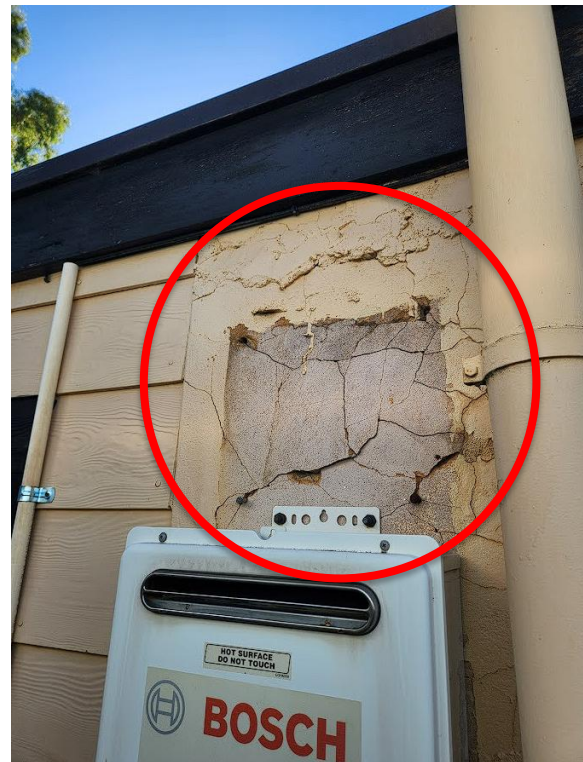
Cracking to render above water heater.
