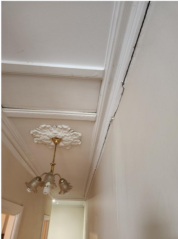
Horizontal cracking to cornice on eastern wall.
