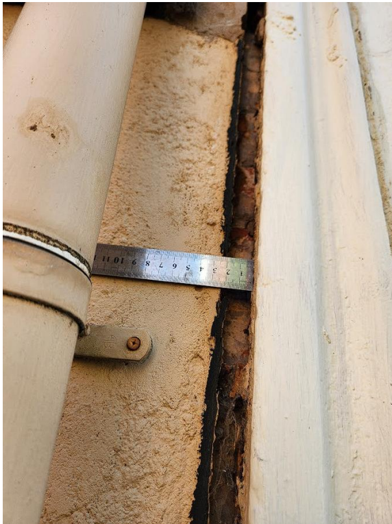
Measurement of separation between render and southern wall.
