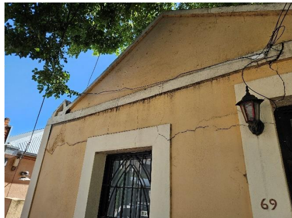
Photo 2 – Cracking in front gable, top of gable leans back towards the applicant's property (opposite to base of wall) creating a "bow" in the wall
