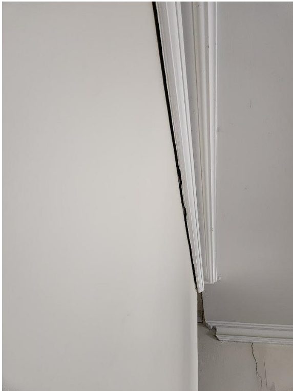
Separation of cornice from northern wall.
