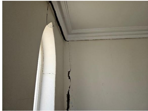
Photo 18 – Western elevation / cornice separation, cracking between western elevation and intersecting internal wall of front lounge room
