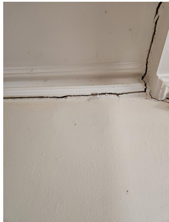
Horizontal cracking to cornice in southeastern corner of corridor.
