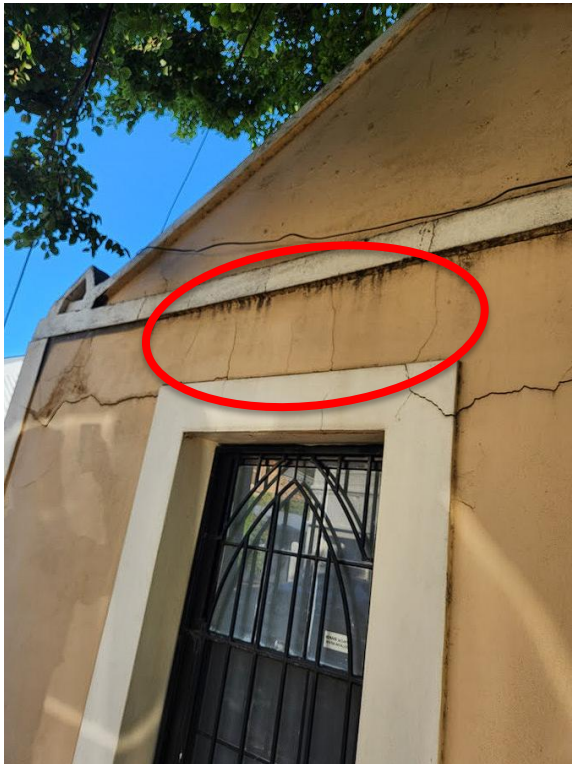
Horizontal and vertical cracking above southern living room window.
