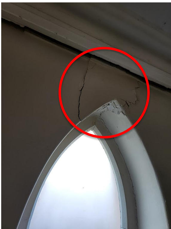
Vertical cracking and debonded render above northern window on western wall.
