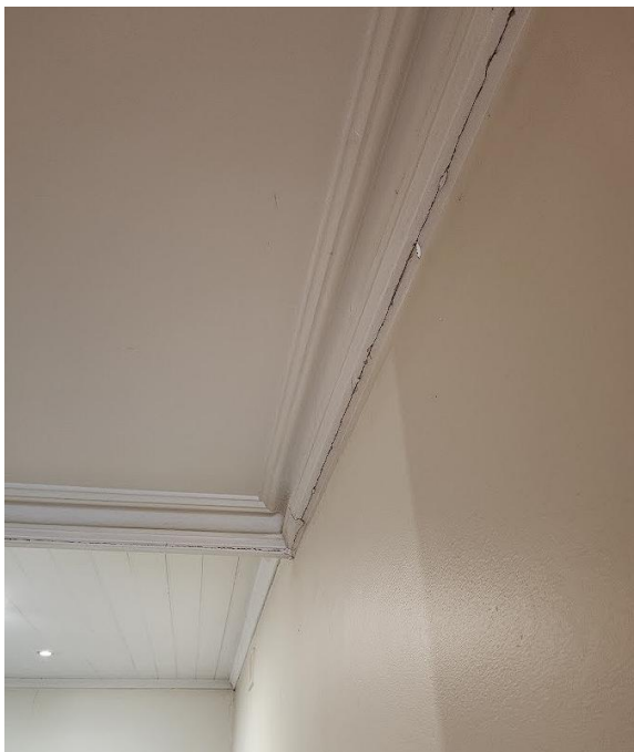
Horizontal cracking at bottom of cornice in northeastern corner of room.
