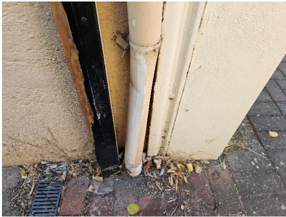
Photo 5 – Railway section positioned against front elevation and assumedly tied through dwelling is indicative of past attempts to stabilise dwelling's front
