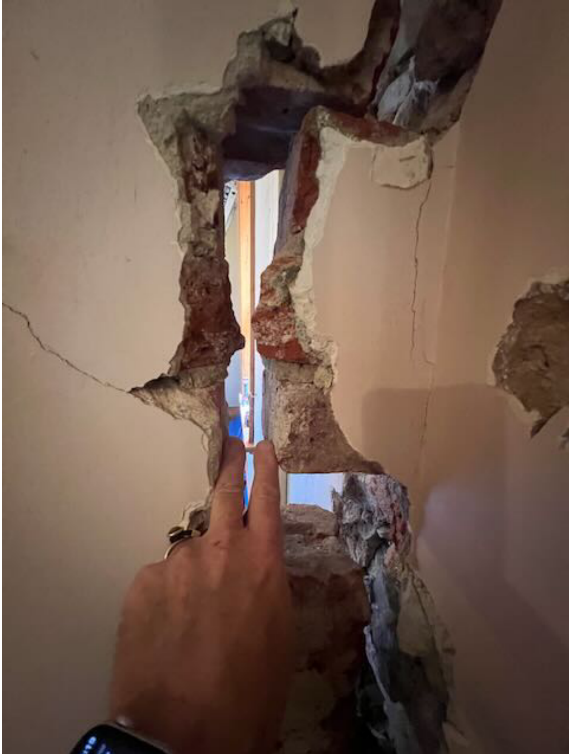
Crack raked out in preparation for side wall being pushed back to plumb.
