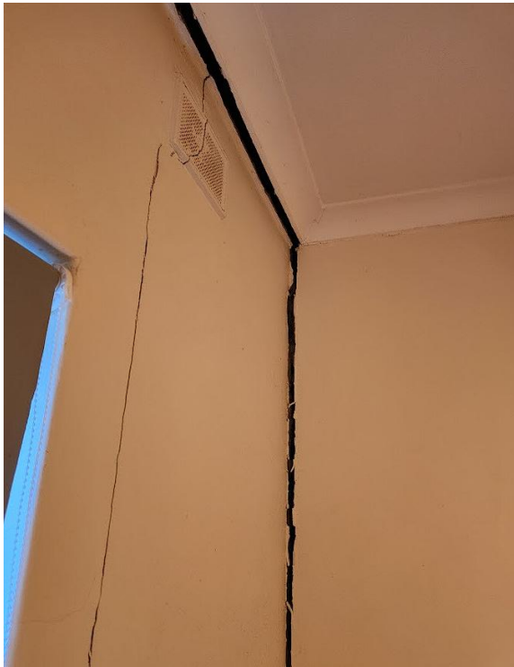
Vertical cracking in northwestern corner of room, indicating rotation of western external wall.
