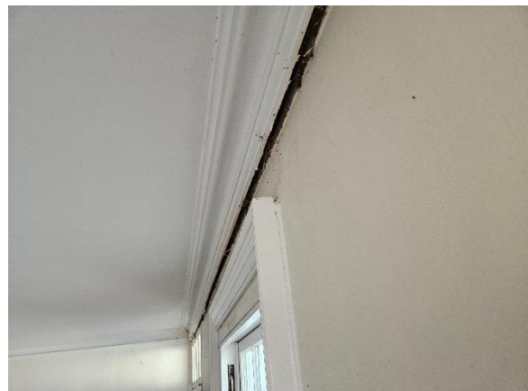
Photo 16 – View of cornice separation along front elevation
