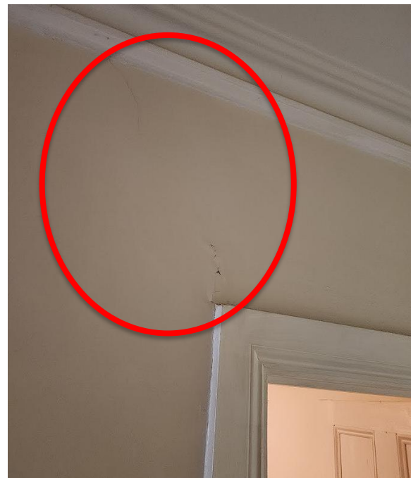
Diagonal cracking above bed 2 door.
