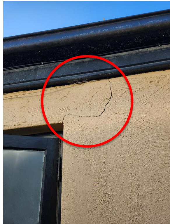
Diagonal cracking above kitchen window.
