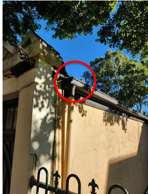
Debris in gutter.
