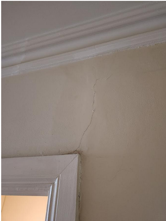
Diagonal cracking above bed 1 door.
