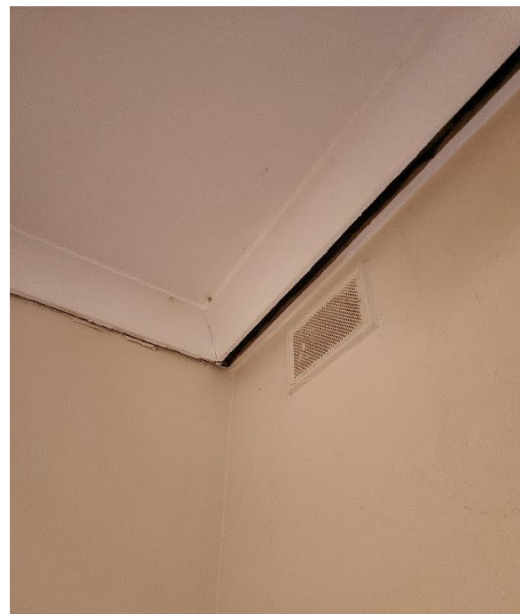
Separation of cornice from western wall on southern end.
