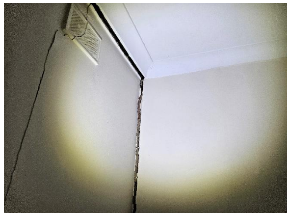
Photo 28 – Separation of bed 1's western wall / cornice, and cracking between western elevation and intersecting wall
