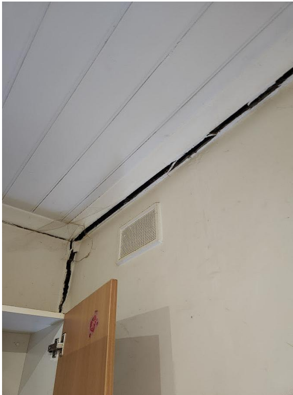
Separation of cornice from western wall, indicating rotation of wall.
