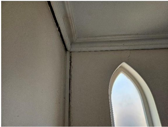
Photo 17 – Broader view of gapping between front elevation and cornice, and at western / front elevation intersection (as shown in closer image in Photo 15)
