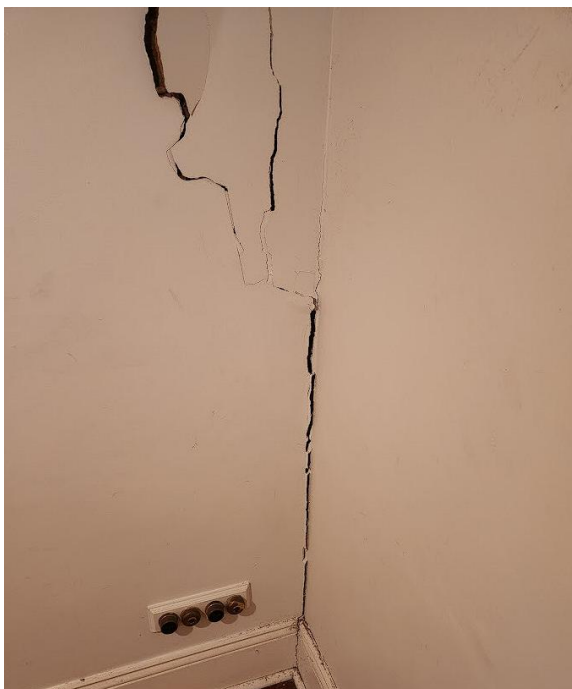
Vertical and diagonal cracking in southwestern corner of room.
