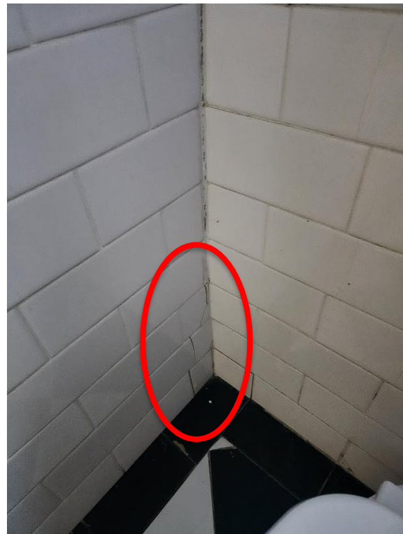
Broken tiles in southwestern corner of room.
