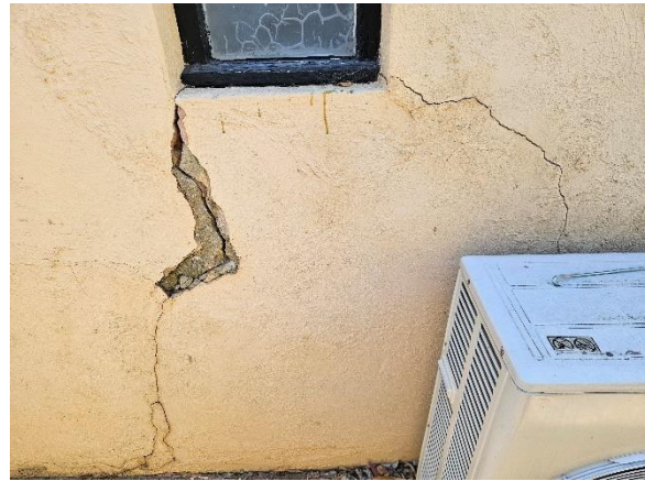
Photo 12 – Example of cracking and previous repair to cracking to western elevation (dislodged render on LHS makes cracking appear more severe)
