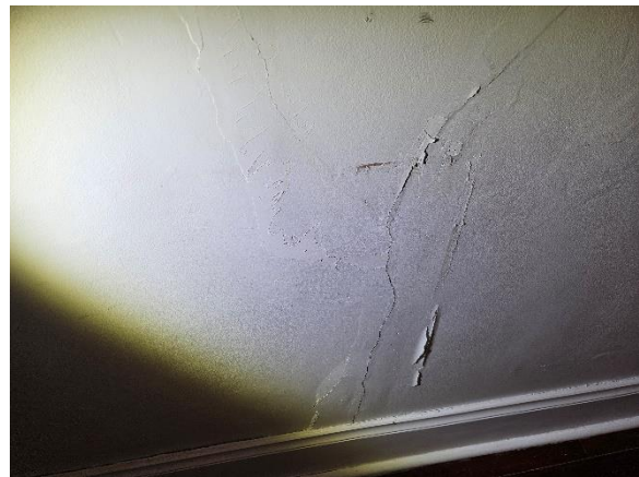
Photo 20 – Example of previous repairs to cracking typically seen to internal walls
