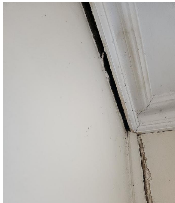
Separation of cornice from southern wall.
