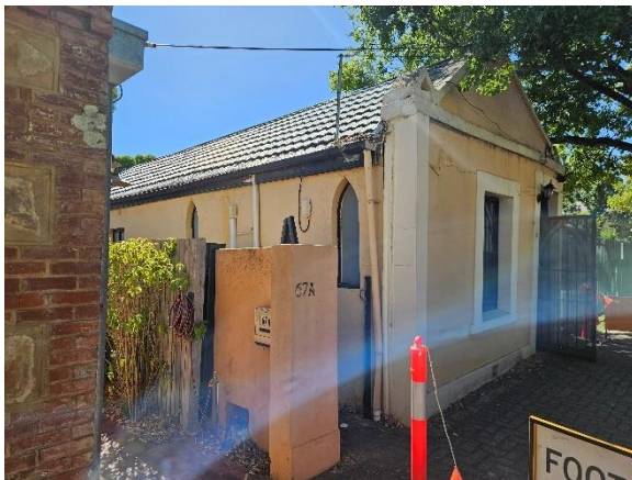
Photo 1 – General view of northern elevation showing lean towards Council footpath and cracking towards top of gable
