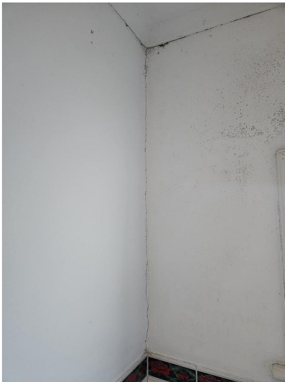
Vertical cracking in southwestern corner of room.
