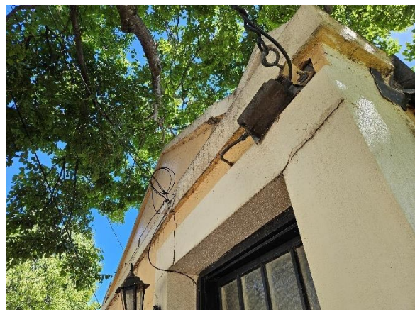
Photo 4 – Cracking at eastern end of front elevation
