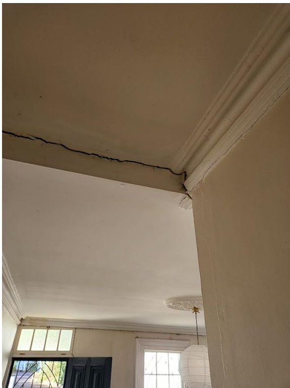
Horizontal cracking to ceiling between lounge room and corridor.
