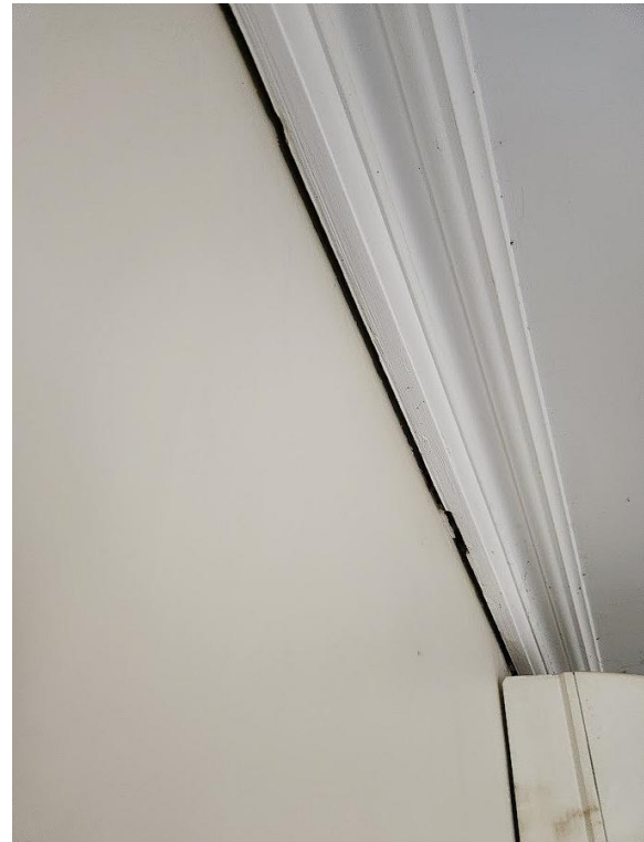
Separation of cornice from western wall.
