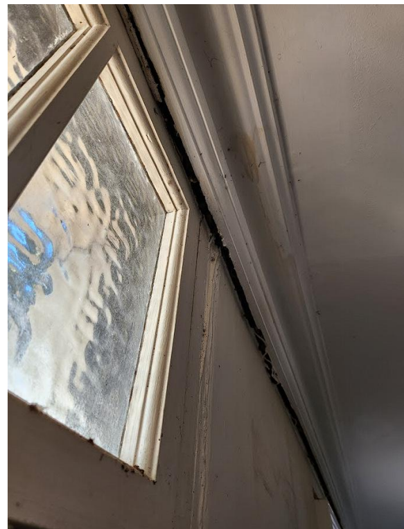
Separation of cornice from southern wall.
