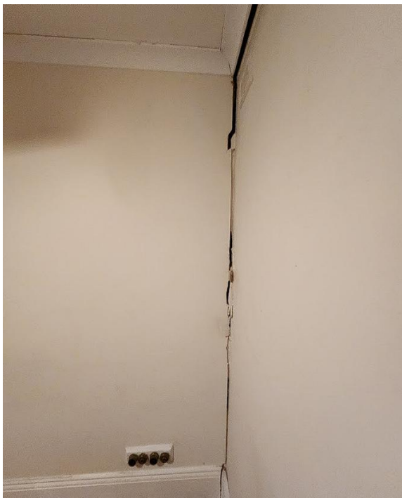
Vertical cracking in southwestern corner of room and separation of cornice from wall.
