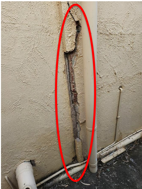
Vertical cracking to external wall near bathroom.
