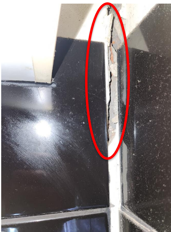
Vertical cracking in southwestern corner of room.
