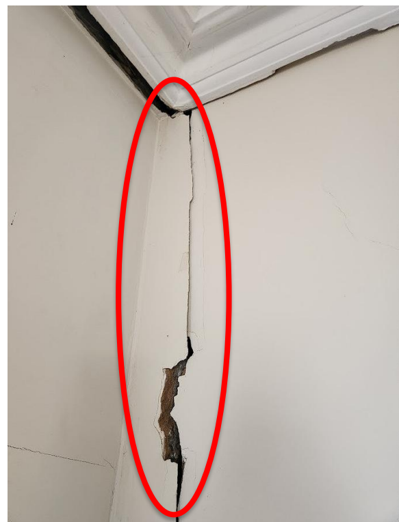
Severe cracking in northeastern corner of room and separation of cornice from wall.
