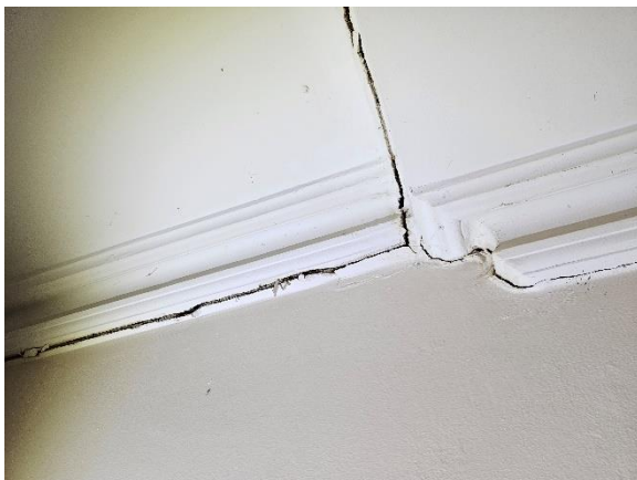
Photo 21 – Example of typical severity of cracking away from area of concern, hallway's eastern wall and cornice / ceiling shown
