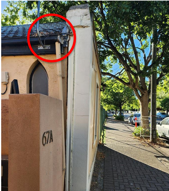
Significant leaning of front wall. Gutter filled with debris.
