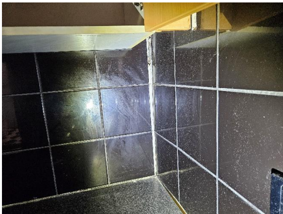
Photo 31 – Tapered vertical cracking in south-western corner of kitchen
