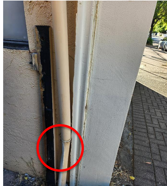
Damaged downpipe and clogged trench drain near side entry door.
