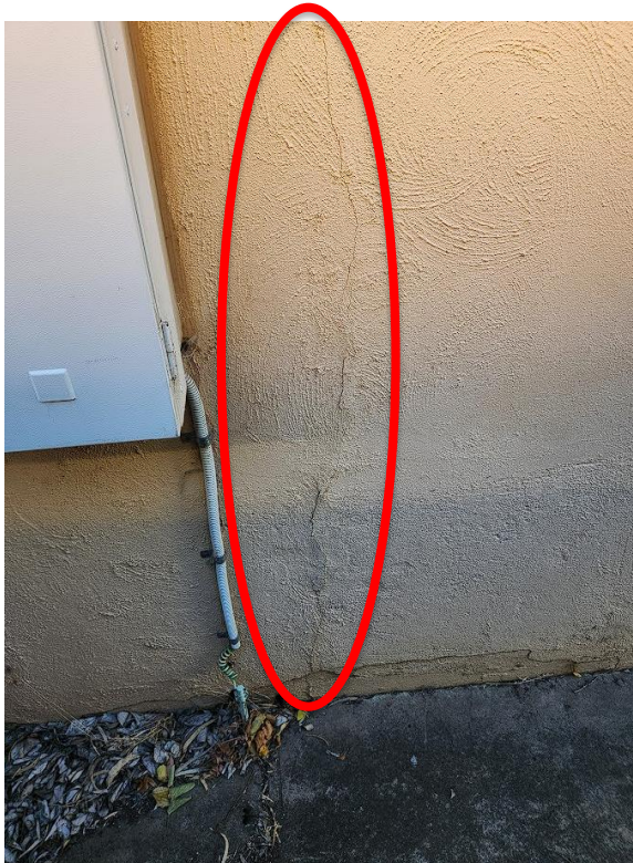
Hairline vertical cracking near meter box.
