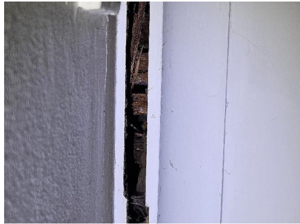
Photo 24 – Close up of separation between bed 1's wall and cornice, showing possible evidence of timber deterioration
