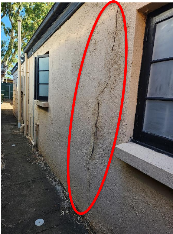
Vertical cracking to the north of bed 2 window.
