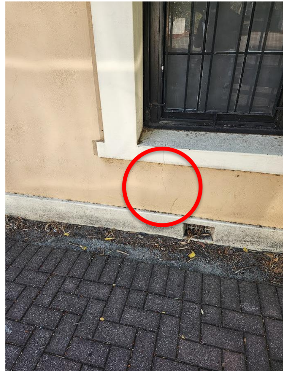
Vertical cracking below southern living room window.
