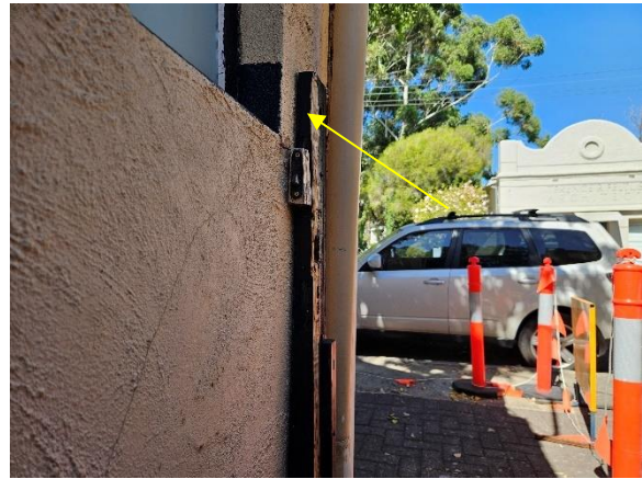
Photo 36 – Tapered wall plate forming part of side gate indicative of past movements to wall (plate thinner at top)
