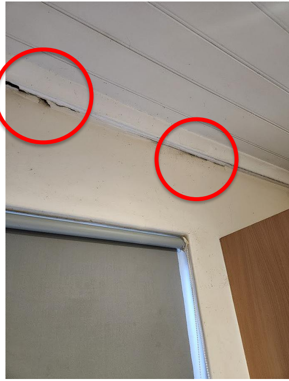
Separation of cornice from western wall was less on northern end.
