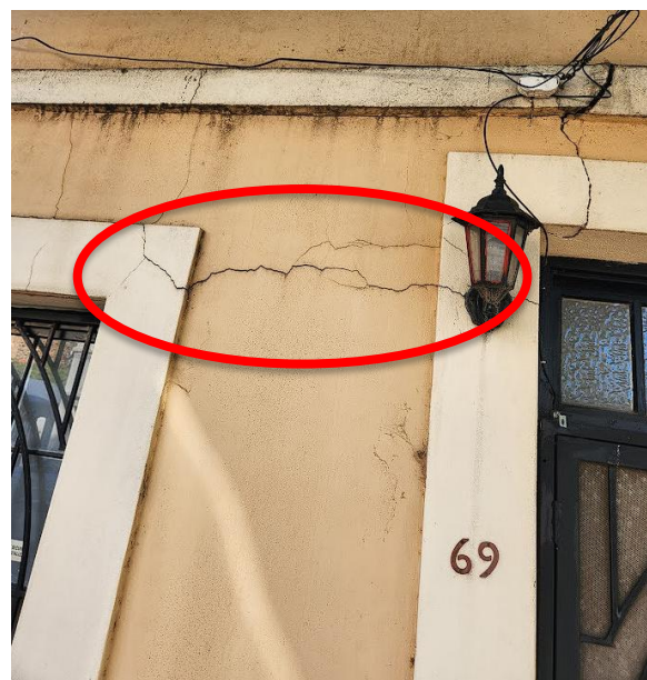
Horizontal cracking west of entry door.
