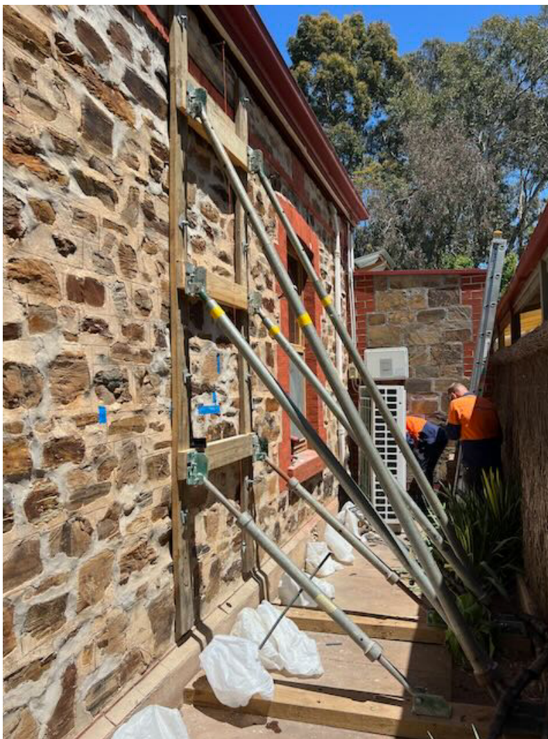
Urathane Solutions undersetting and straightening wall
