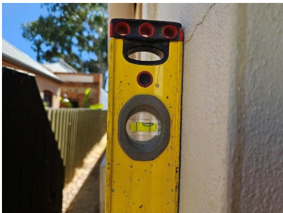
Photo 9 – Spirit level placed against southern end of western elevation showing outward lean towards the adjacent property
