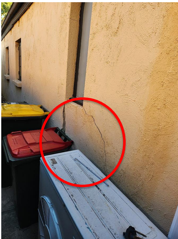
Diagonal cracking and debonded render near air conditioning unit.
