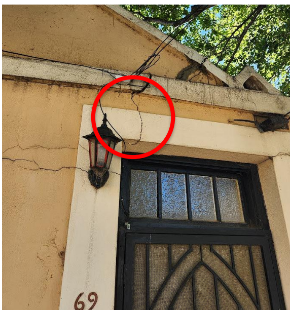
Vertical cracking above entry door.
