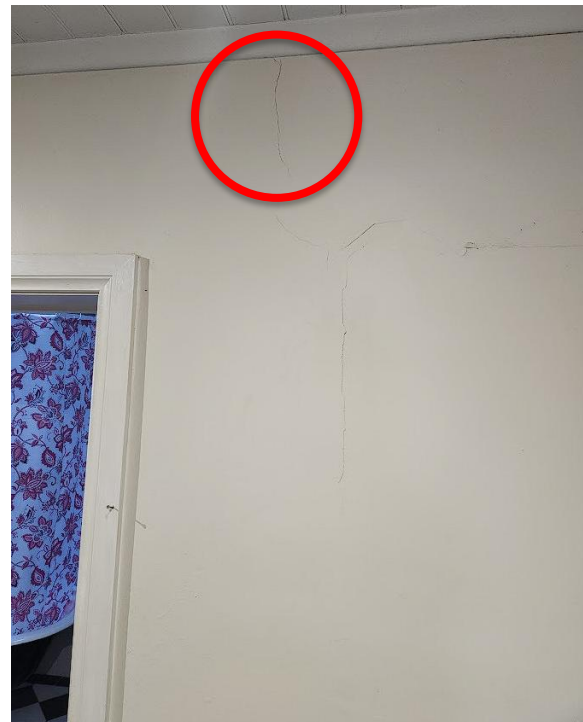
Vertical cracking to northern wall of room.
