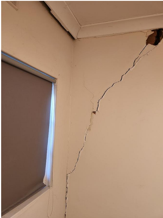
Diagonal cracking to northwestern corner of room.
