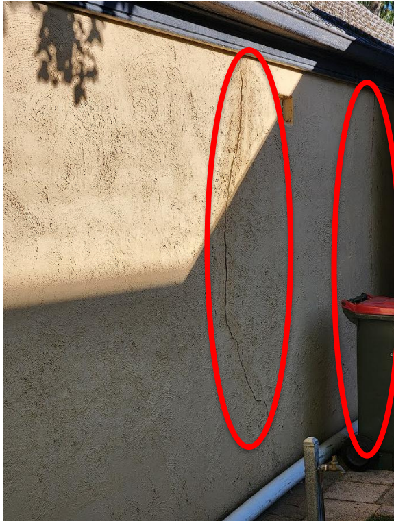
6-7mm diagonal cracking and 3-4mm vertical cracking on eastern boundary wall (from childcare side).
