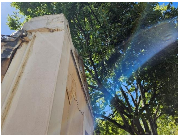
Photo 3 – Side view of top of gable attempting to capture horizontal bow in wall
