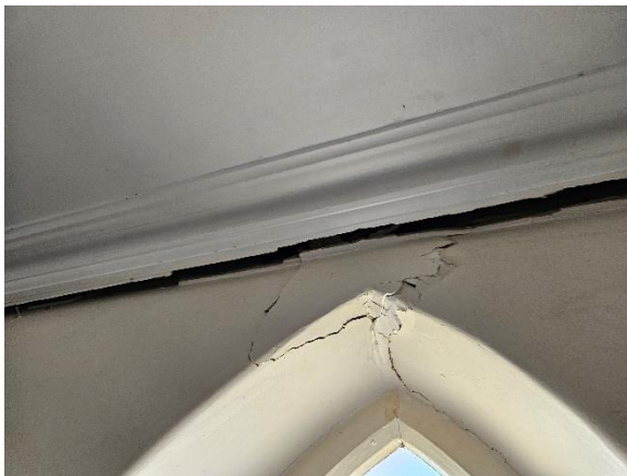
Photo 19 – Cornice separation along western wall, previous crack repairs and recent cracking above window
