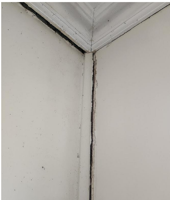
Vertical cracking and separation of cornice in southwestern corner of room.
