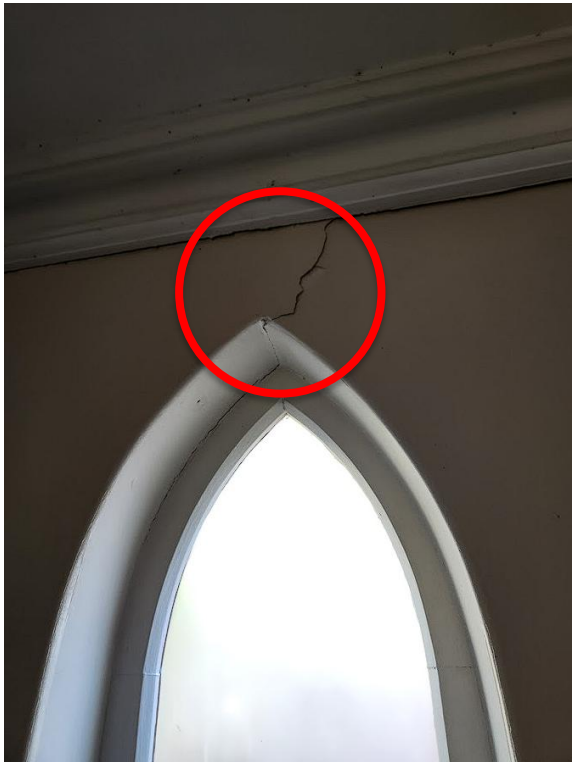
Diagonal cracking above southern window on western wall.
