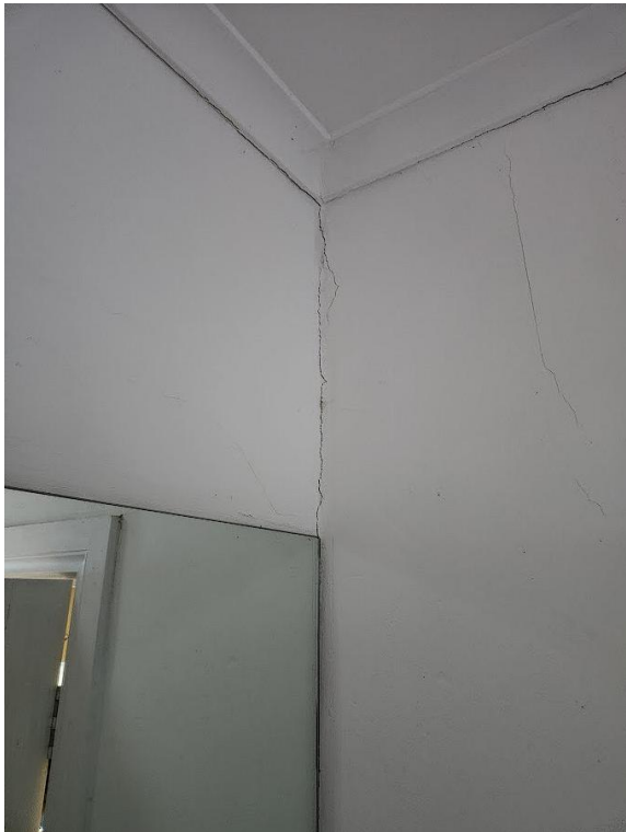
Vertical cracking in northeastern corner of room.
