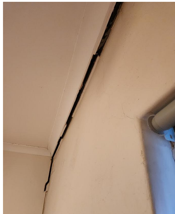
Separation of cornice from wall.
