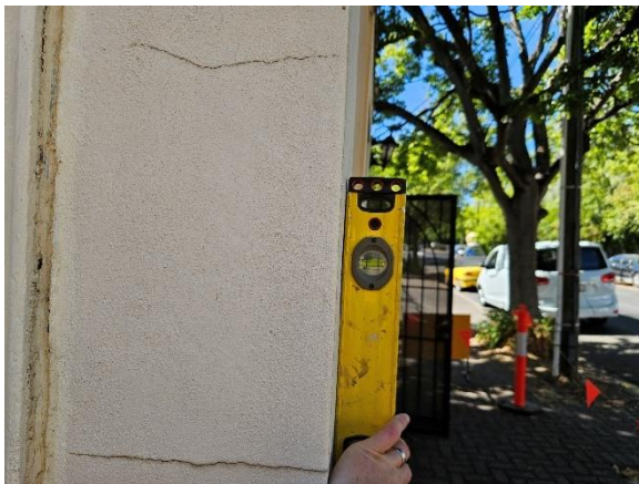
Photo 7 – Spirit level placed against front elevation showing lean towards footpath
