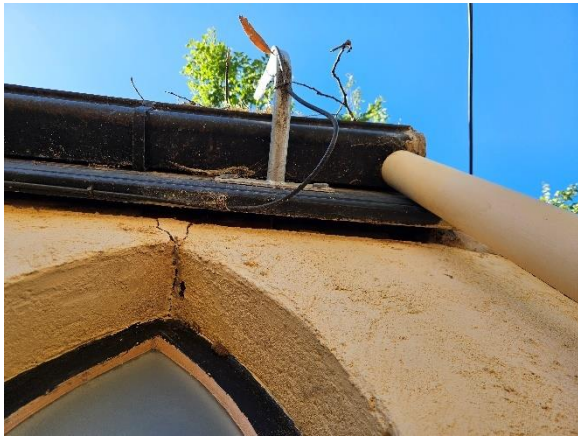
Photo 11 – Separation between western elevation and fascia
