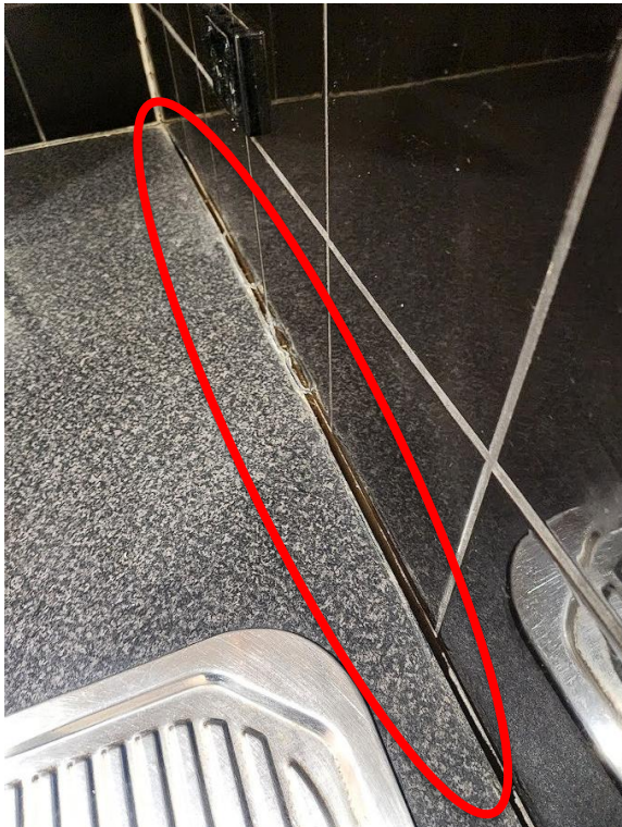
Separation of kitchen benchtop from western wall, indicating rotation of wall.
