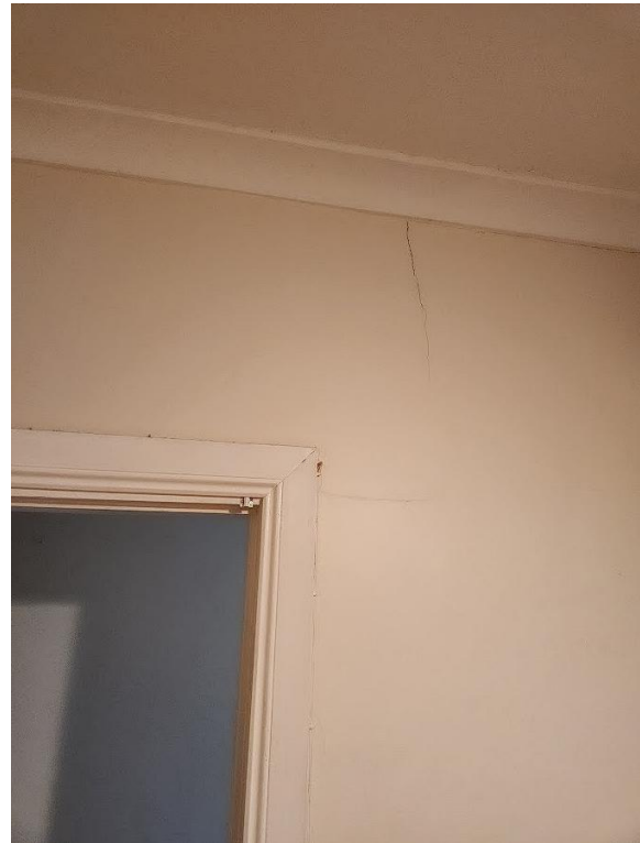
Vertical cracking above door.
