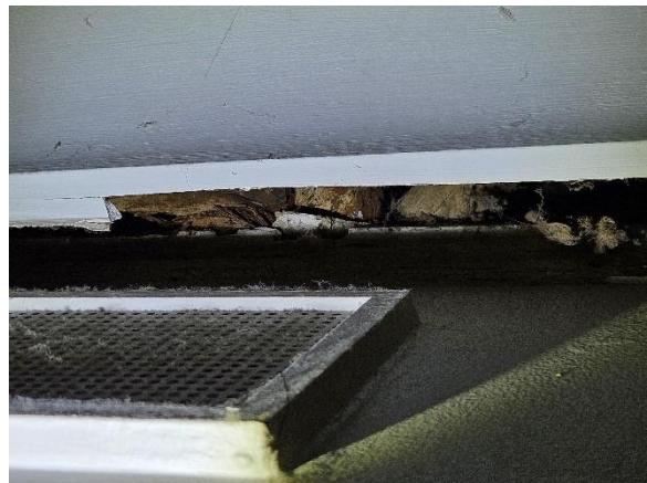
Photo 26 – Separation and missing filler showing possible evidence of timber deterioration
