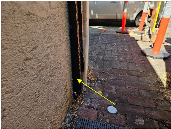
Photo 35 – Tapered wall plate forming part of side gate indicative of past movements to wall (plate thicker at bottom)
