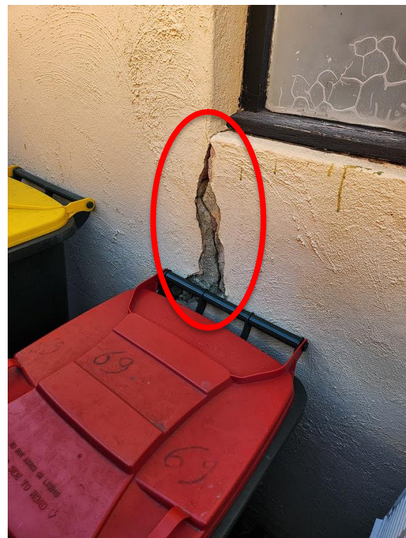
Vertical cracking below northern lounge room window on western wall.
