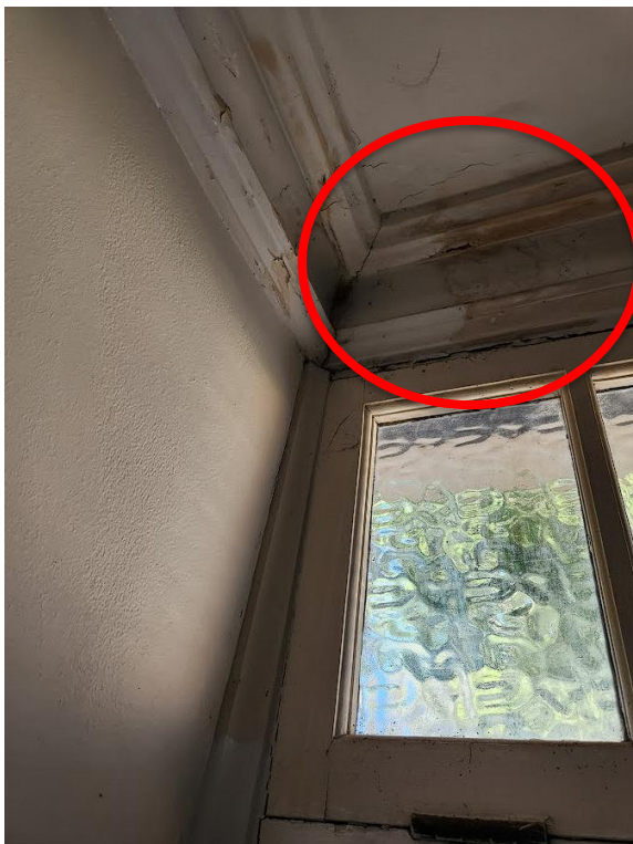
Water damaged in southeastern corner of room, above entry door.
