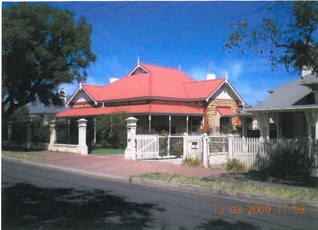
Trinity Gardens Photo 3: Example of return verandah villa of freestone construction.
