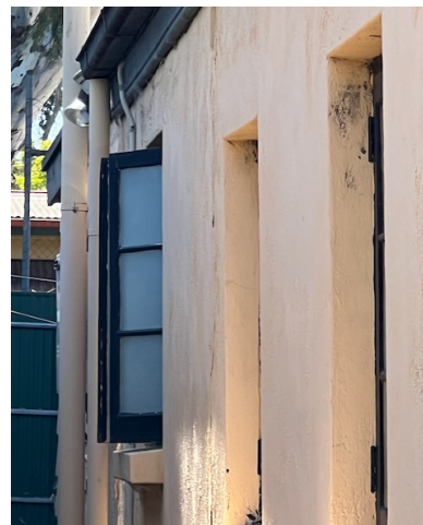
Original casement windows
