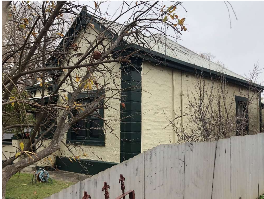
13. Adjacent villa of similar construction with steel restraining posts. Good condition
