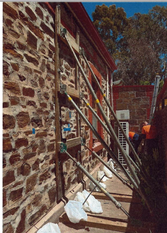
Pushing whole side wall back to plumb. Cost $20K
