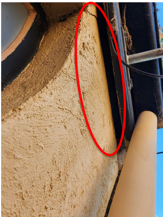
Separation of fascia from wall near southwestern corner of building.
