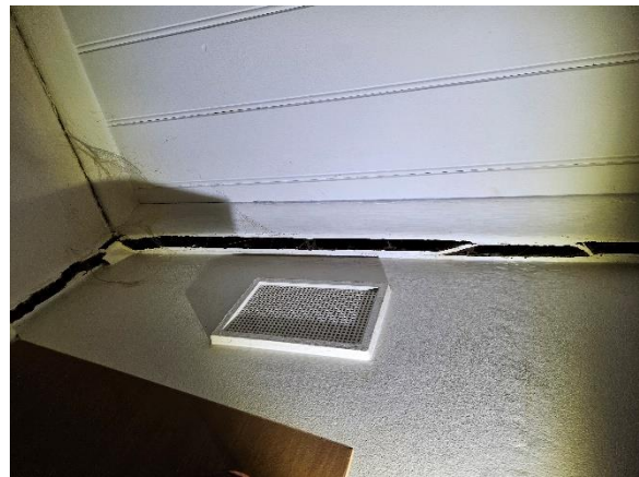
Photo 32 – Top of cracking shown in Photo 31, as well as separation of the western wall / cornice junction (including previous filling material)
