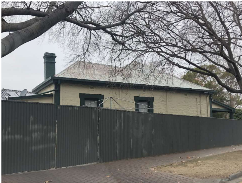
14. Adjacent villa of similar construction with steel restraining posts. Good condition
