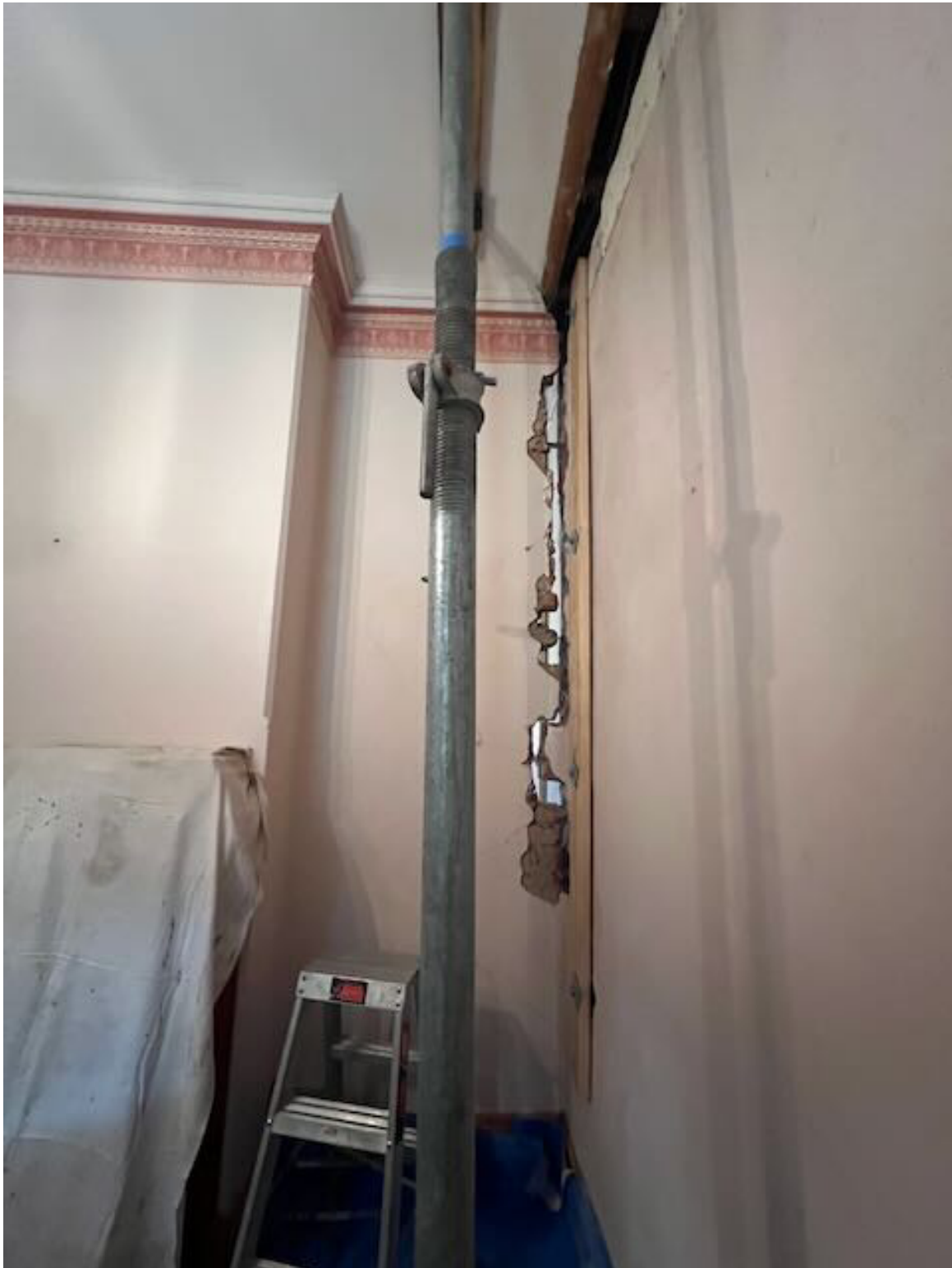
Crack raked out in front room in preparation for side wall being pushed back to plumb.
