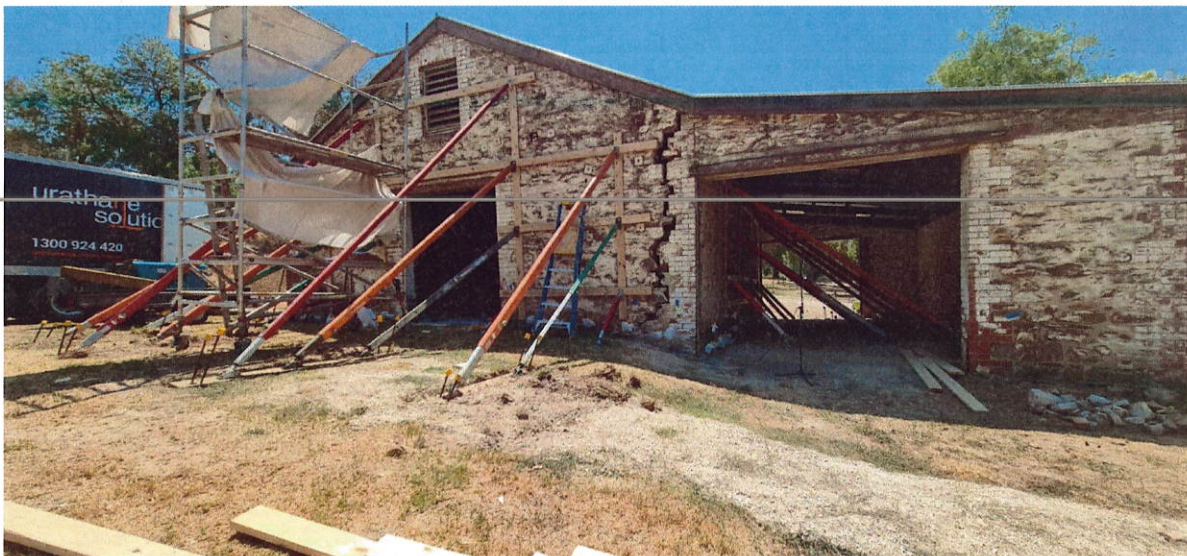
Urathane Solutions repairing wall in Dawesley, Adelaide Hills
