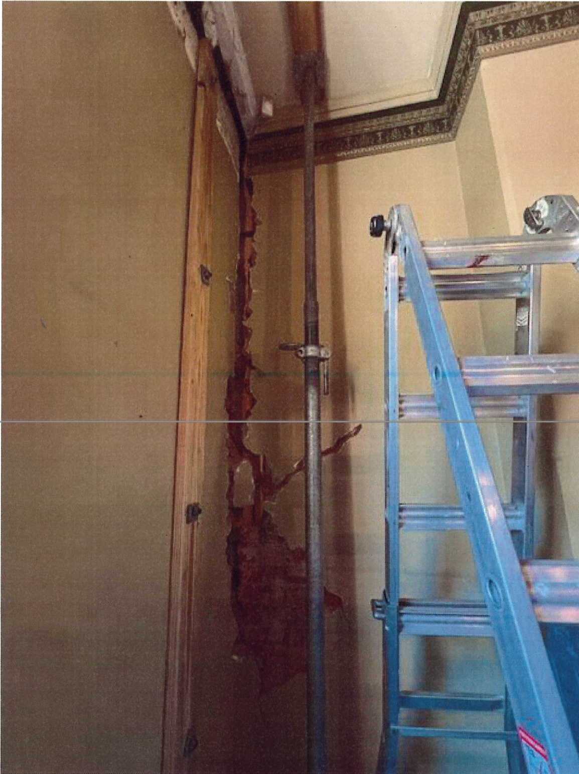
Crack raked out in second room in preparation for side wall being pushed back to plumb.
