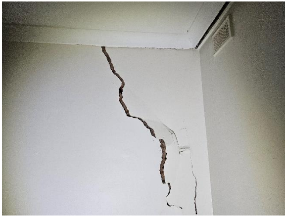
Photo 29 – Cracking to bed 2's southern wall near intersection with western wall, note also separation of western wall / cornice junction
