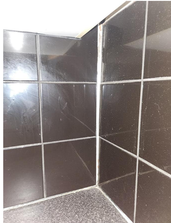
Separation in southwestern corner of room, indicating rotation of wall.
