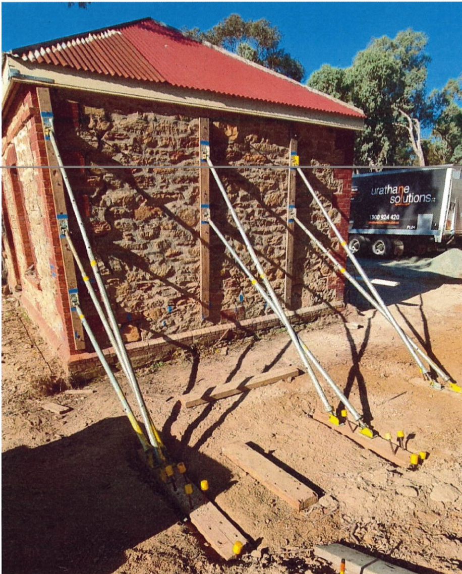
Urathane Solutions pushing wall back to plumb in Oakbank
