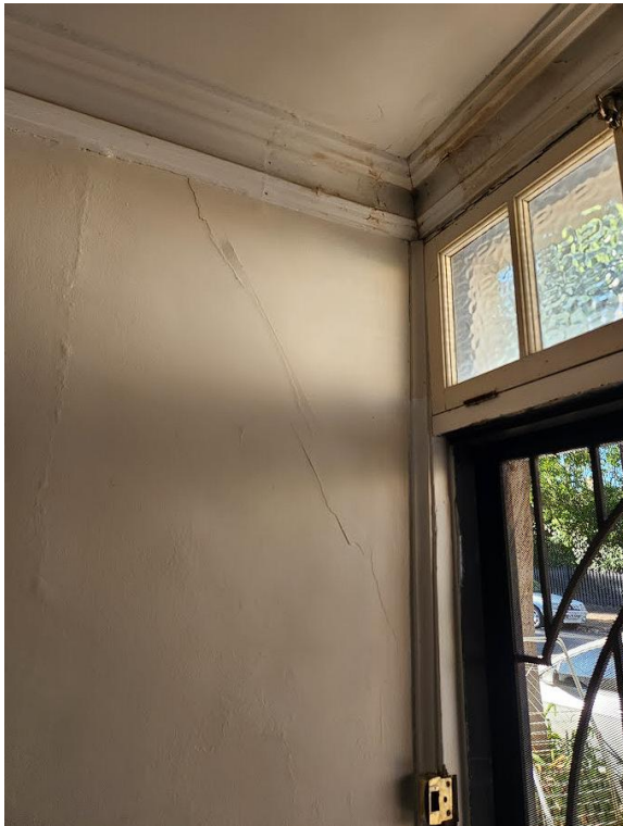
Diagonal cracking on eastern wall, near entry door.
