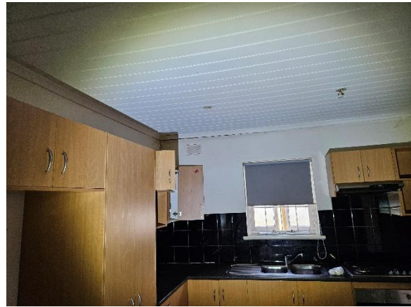
Photo 30 – General view of the kitchen area
