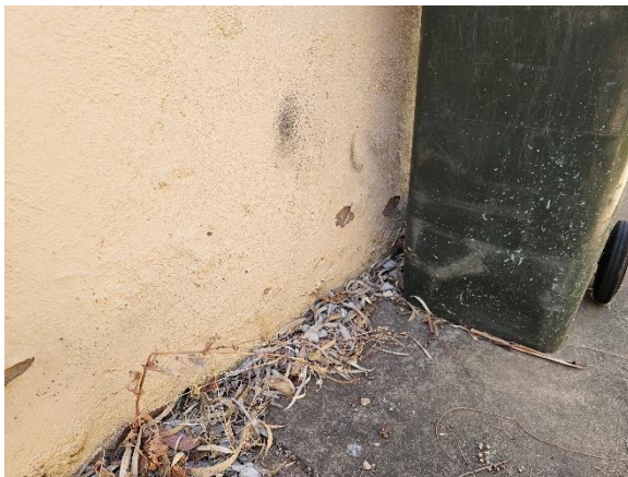
Photo 13 – Bubbling / blistering of lower paint finish along western elevation indicative of rising damp
