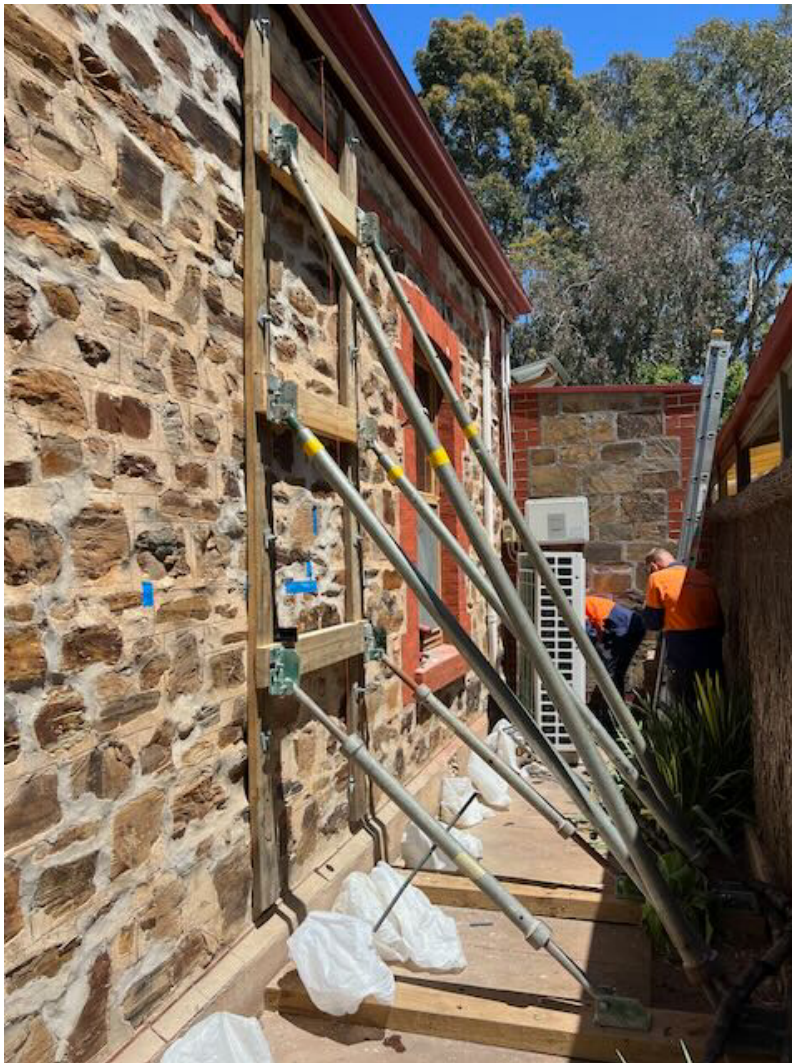
Urathane Solutions undersetting and straightening wall
