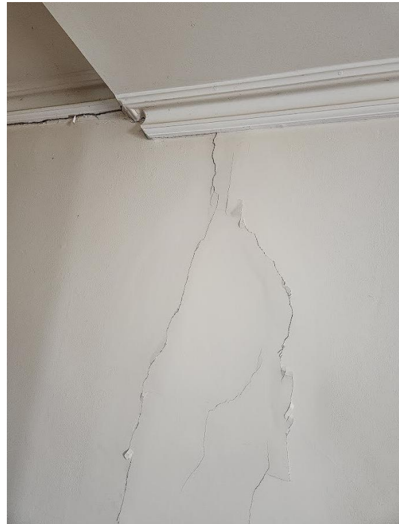
Vertical and diagonal cracking on eastern wall of lounge room.
