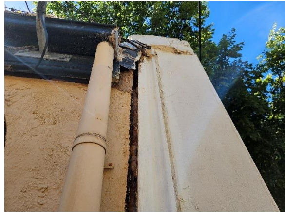
Photo 6 – Tapered separation between railway section and front elevation indicative of worsening in external wall rotation over time
