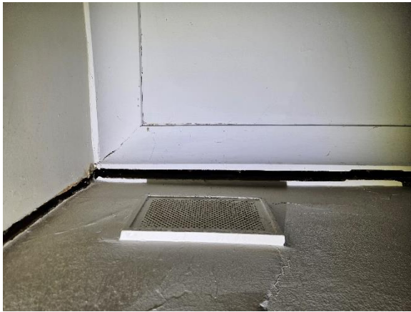
Photo 23 – Separation at bed 1's western wall / cornice junction and intersecting wall
