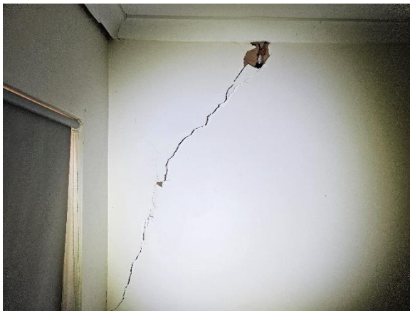
Photo 25 – Cracking to bed 1's northern wall, dislodged of plaster at top of wall makes cracking appear more severe, note also separation of western wall/cornice visible
