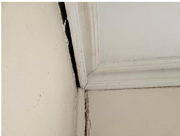
Photo 15 – Gap between front elevation and cornice as well as previous filling, note also separation between corner beading and wall – beading evidence of past attempts to conceal gapping at this wall junction
