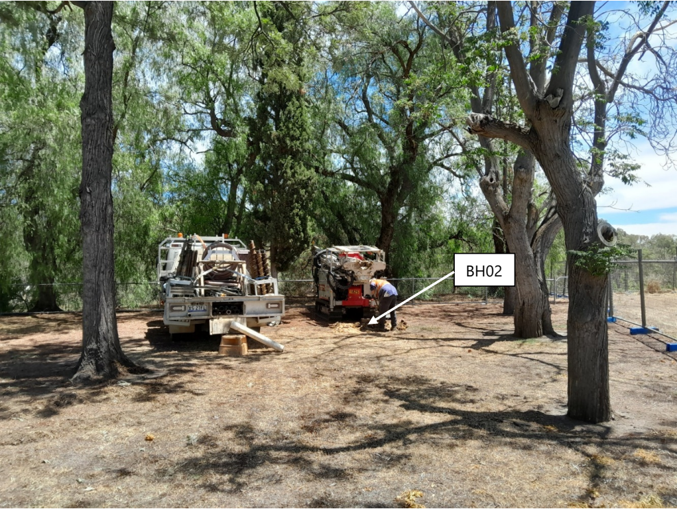
Figure 5: Borehole BH02 location
