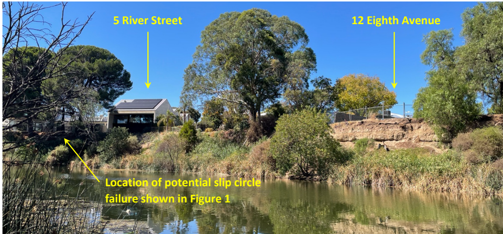
Figure 2. Current state of St Peters Billabong embankment.
