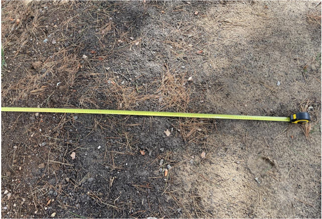
Photo 3.2 Tension crack filled (photograph taken 28 May 2025)
