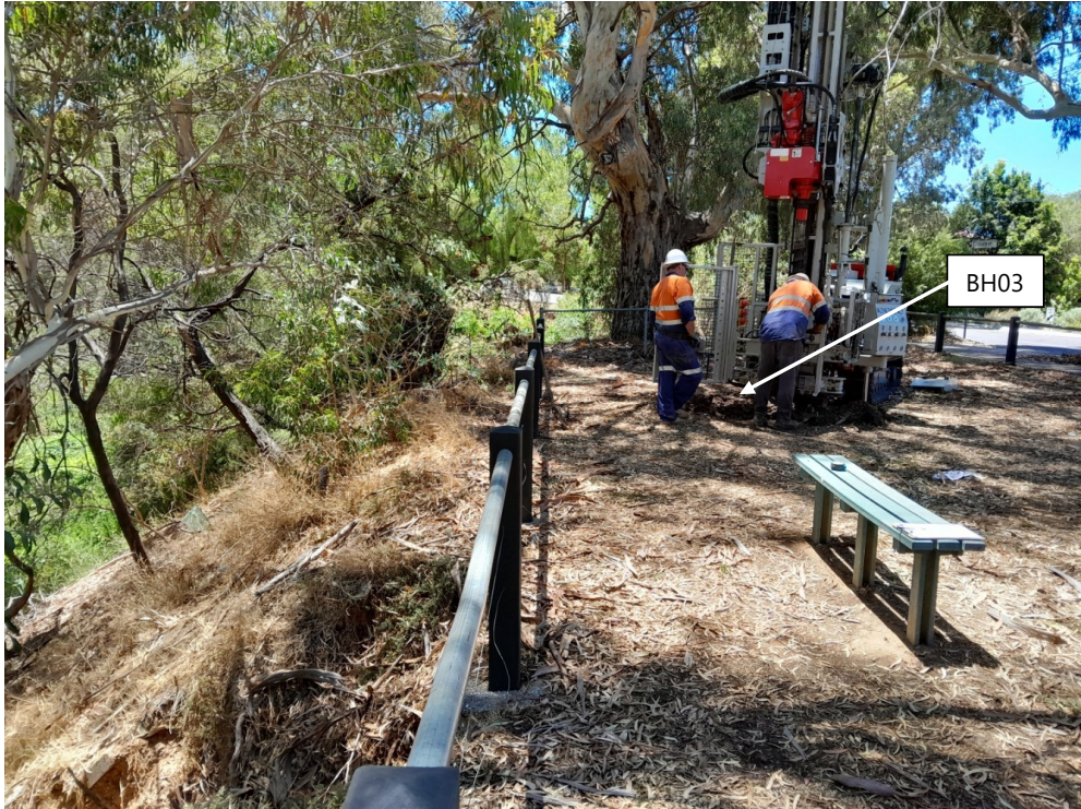
Figure 6: Borehole BH03 location
