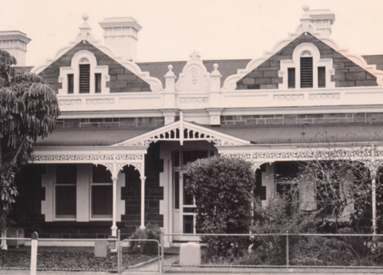
6. Historic Terrace Houses
