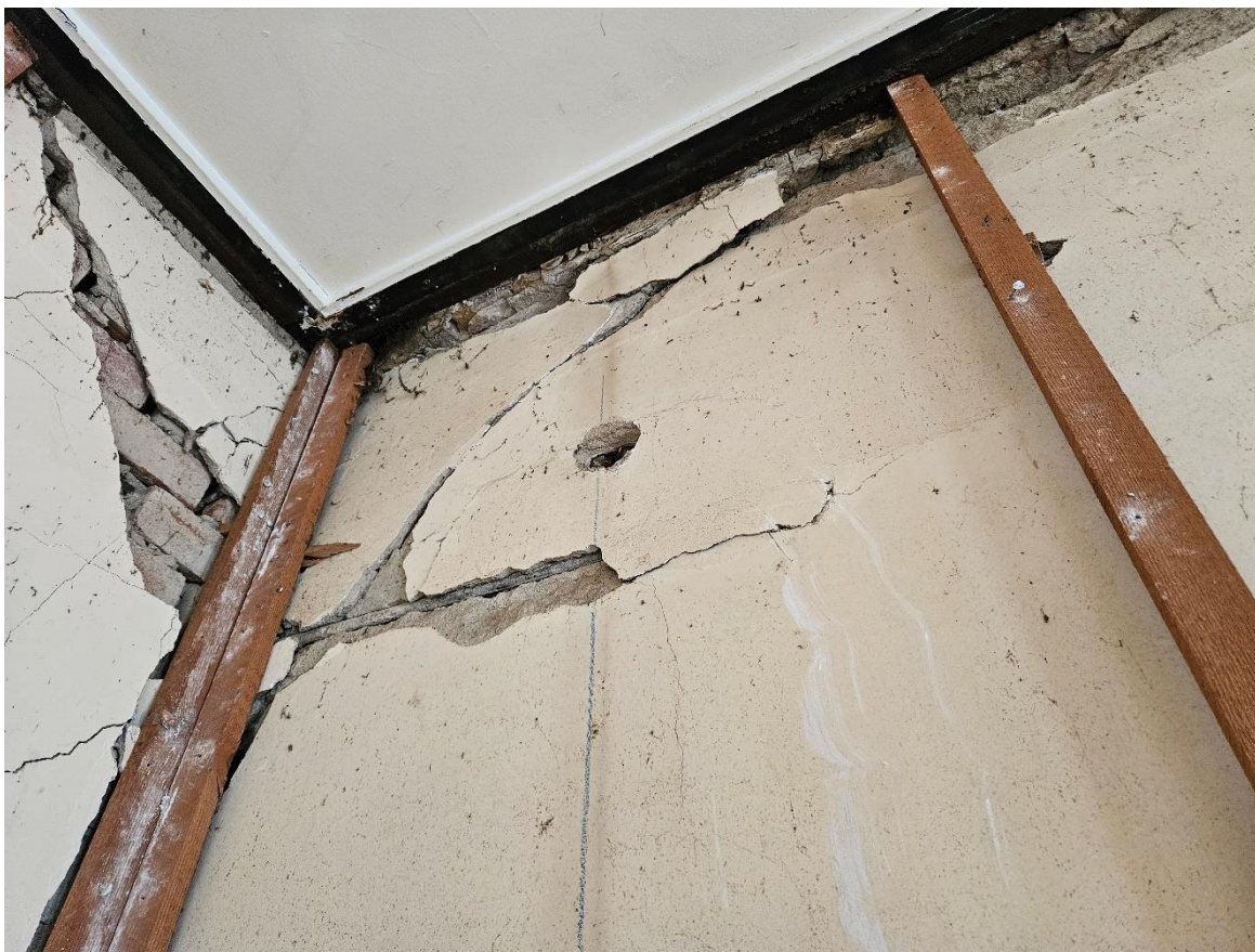
Photo 7 – Tie-rod chased into northern wall of Bed 1, distortion to walls and deterioration of plaster
