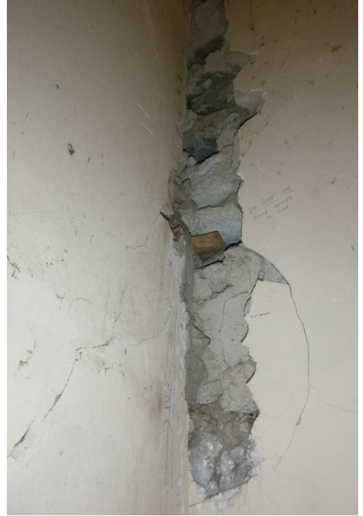
Exposed random rubble construction – Bedroom 1
