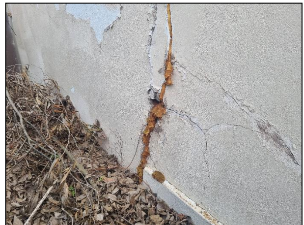
Photo 9 – Structural cracking to southern external wall with evidence of prior gap filling (inadequate)
