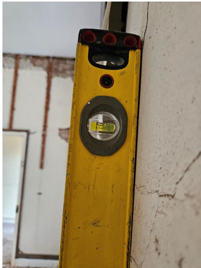
Photo 12 – Rotation of Bed 2's eastern wall consistent with long-term settlement towards east
