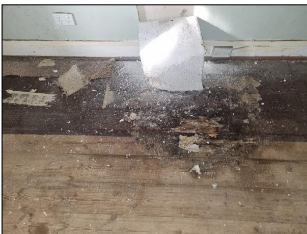
Photo 12 – Moisture damage to timber floorboards due to roof leak above
