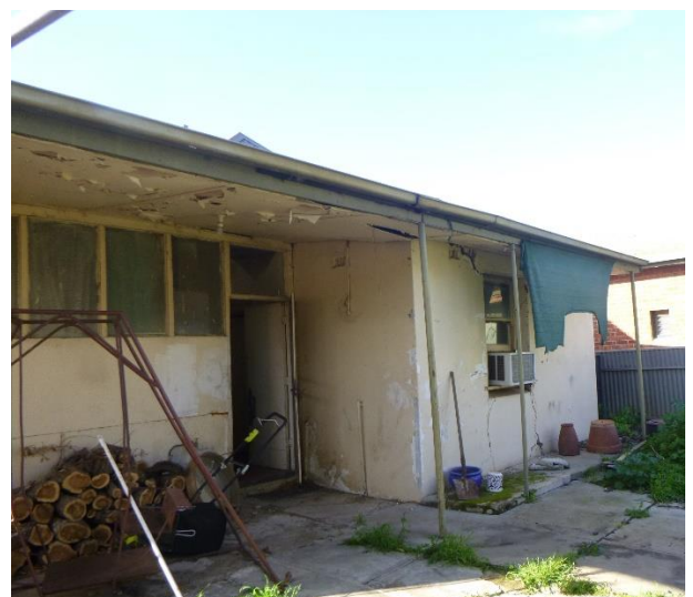
Lean-to construction at rear
