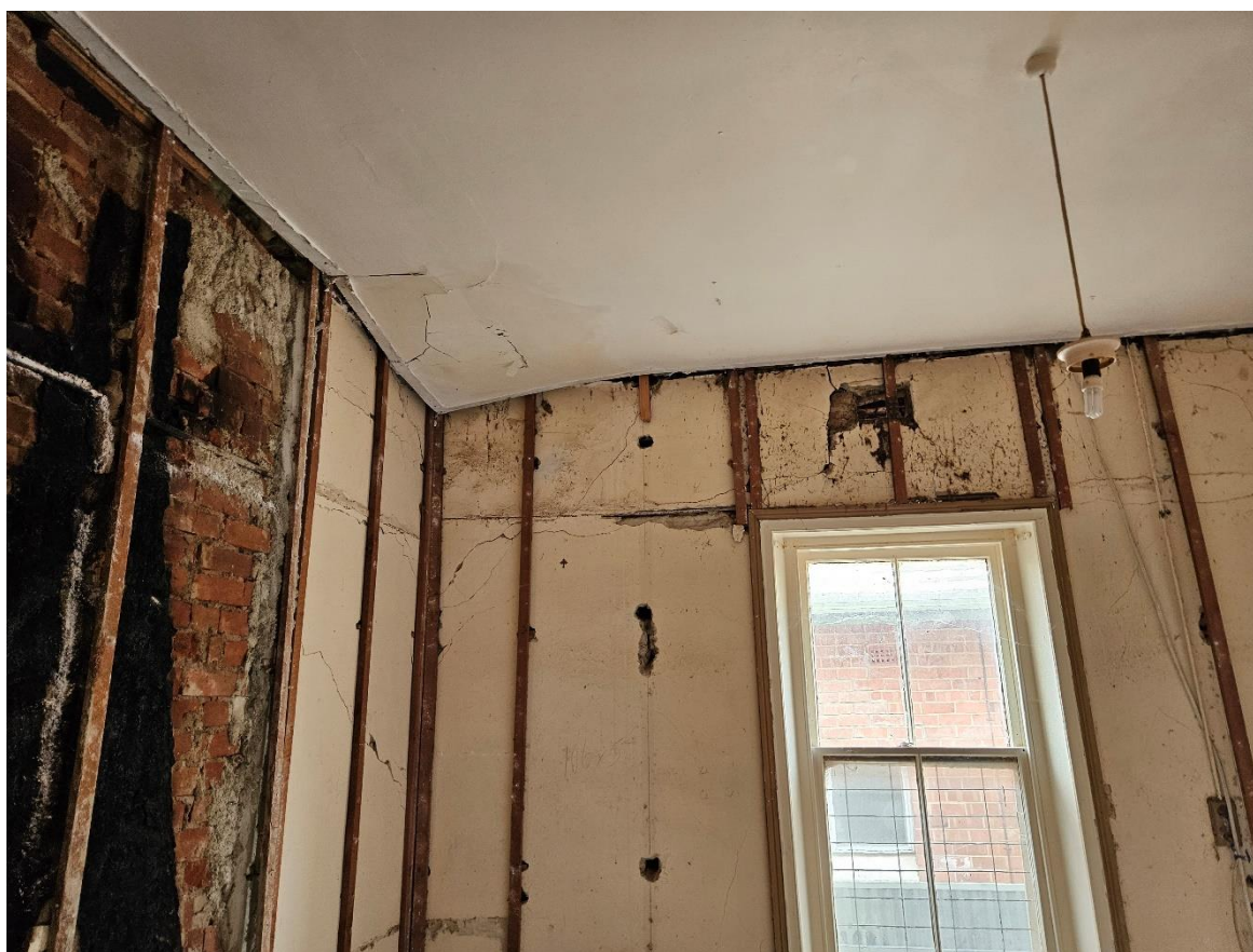
Photo 13 – Living room's ceiling has detached from frame in south-eastern corner
