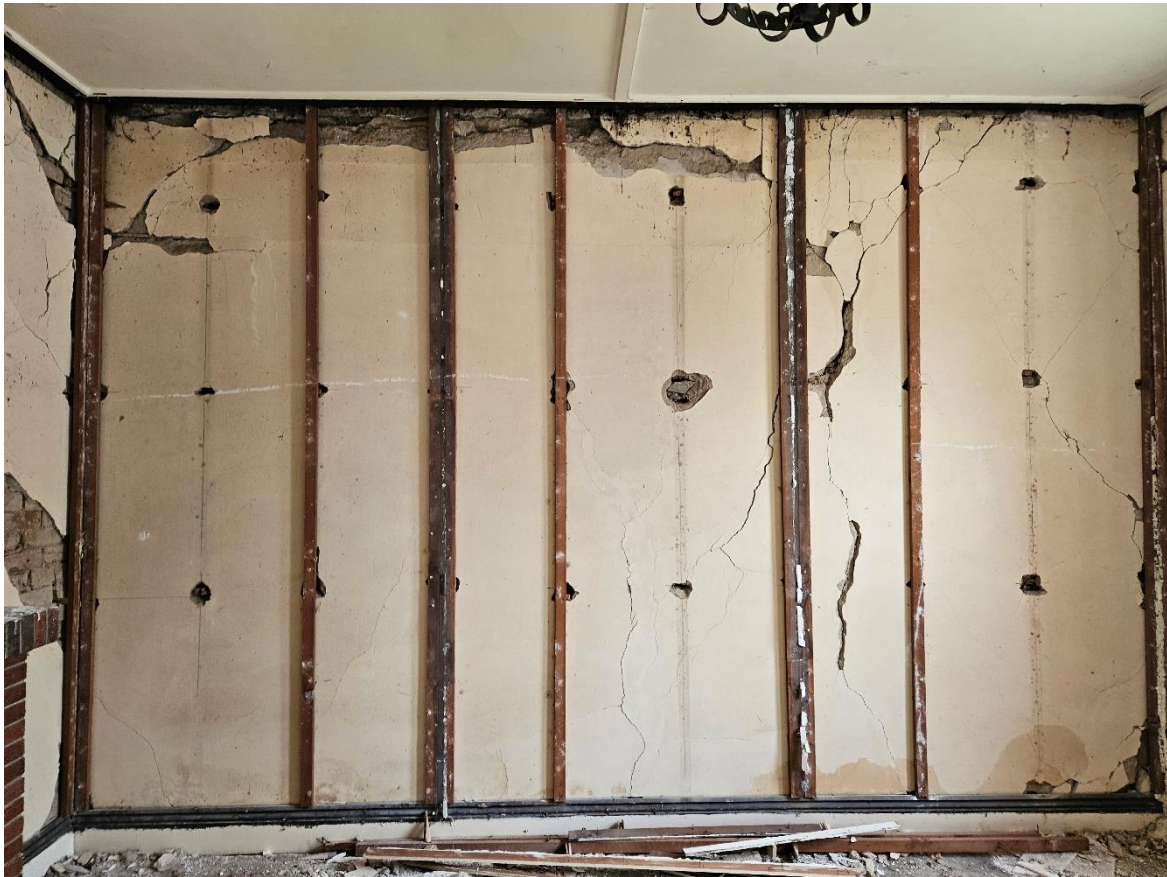
Photo 3 – Bed 1's northern wall
