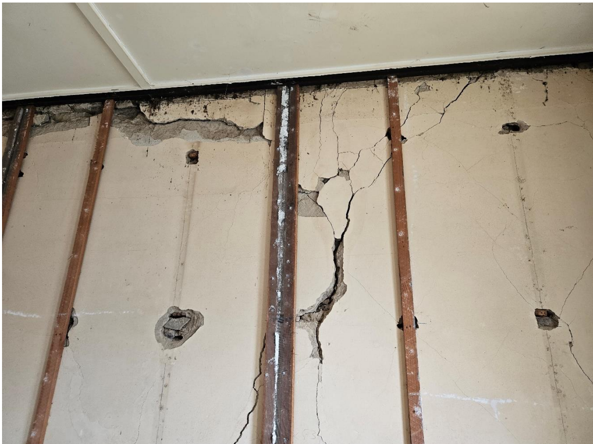
Photo 4 – Bed 1's northern wall
