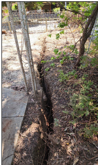
8.3 mtr long by 600 mm deep trench to driveway and car port edge.
