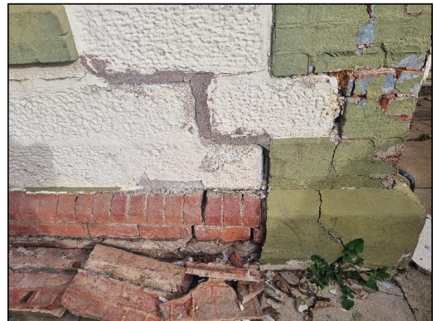
Photo 7 – Structural cracking to northern eastern external walls with evidence of prior crack filling
