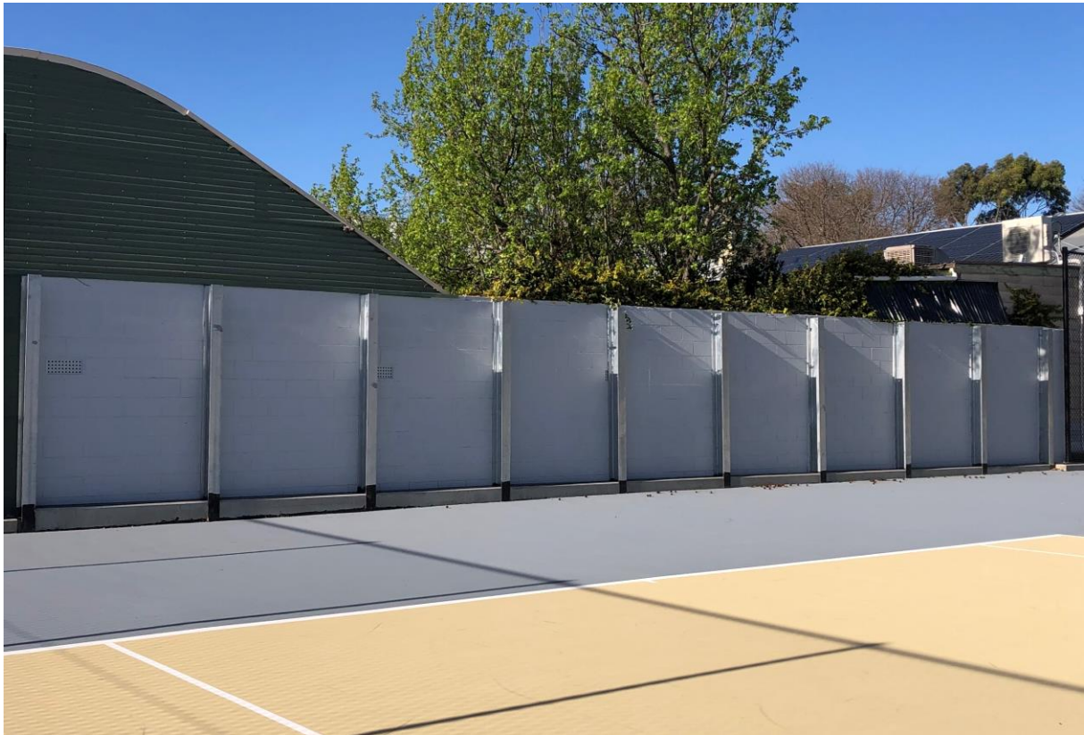
Figure 1: Wall at the north-western end of Burchell Reserve, St Peters, adjacent to the multipurpose courts
