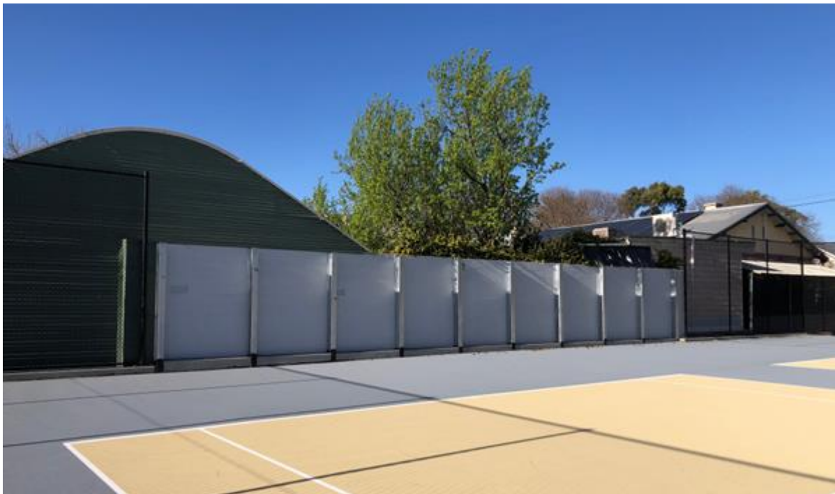
Figure 2: Wall at the north-eastern end of Burchell Reserve, St Peters
