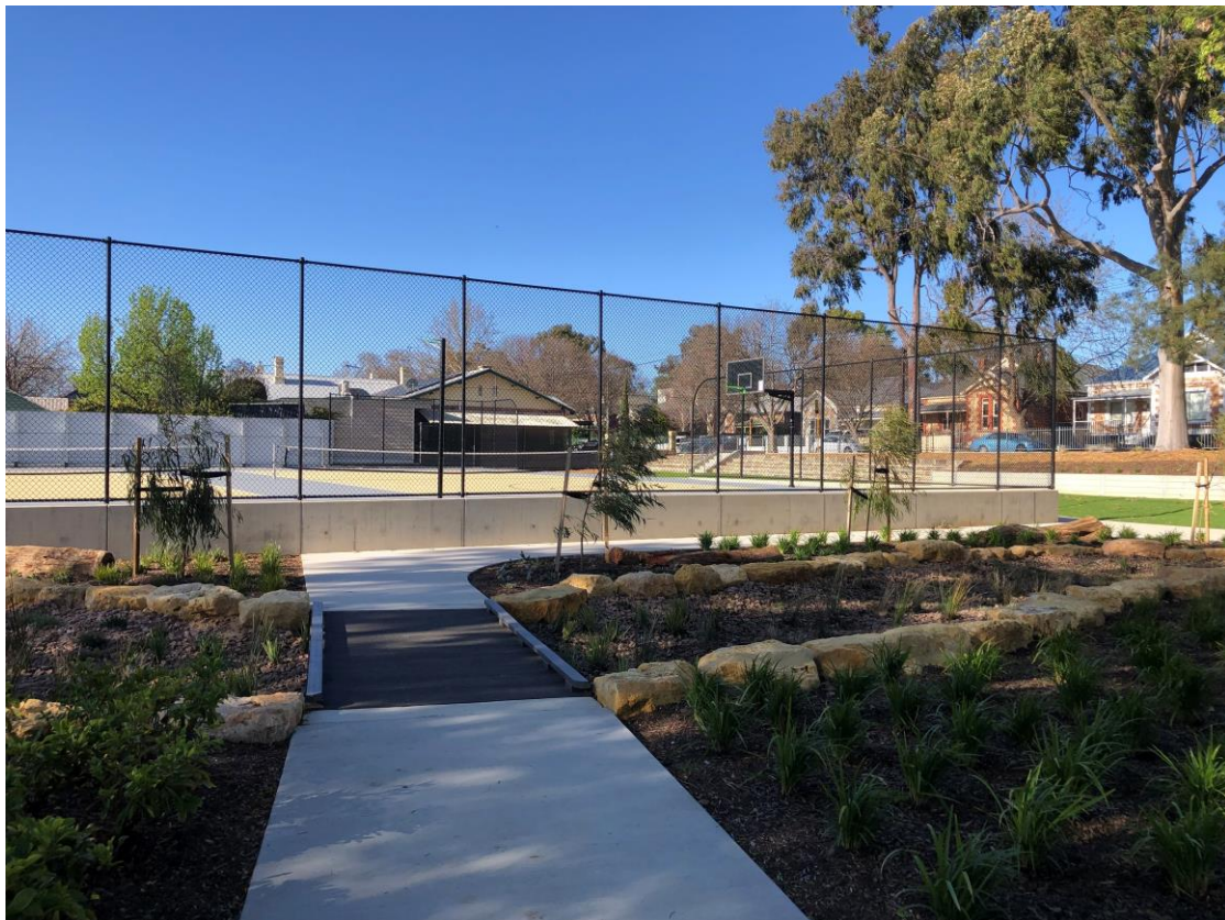
Figure 3: Pathway leading to the multipurpose courts showing retaining wall
