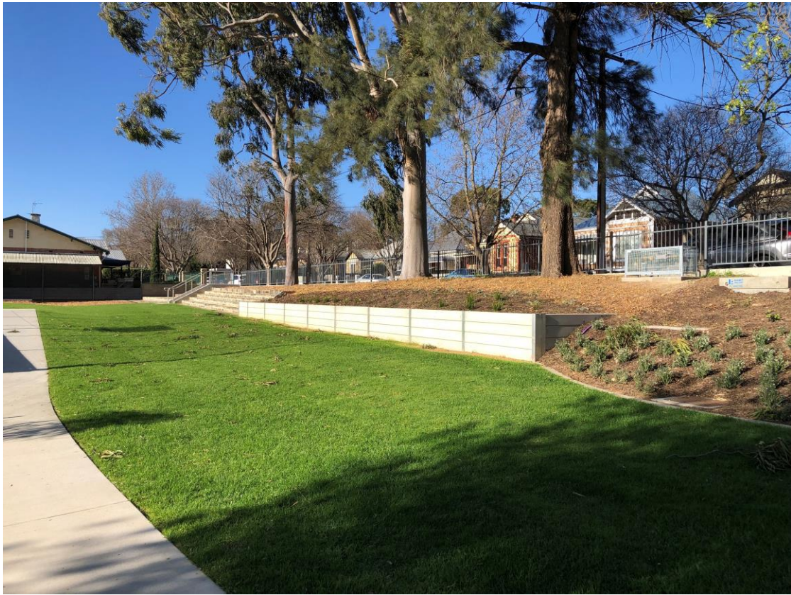
Figure 4: Retaining wall adjacent to Sixth Avenue
