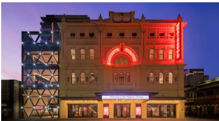
$66 million redevelopment of the 1913 HMT on Gouger St where patron facilities have been pushed out into the newly build section of the theatre.
