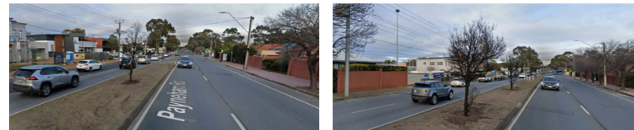
Remove failing trees and box out larger area to support healthy growth of new planting
