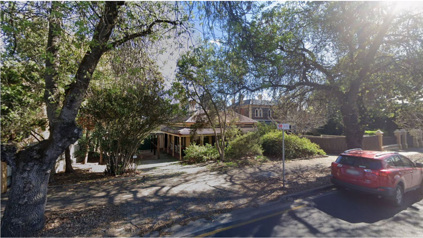
VIEW FROM FLINDERS STREET - LOOKING NORTH-EAST - BEFORE
