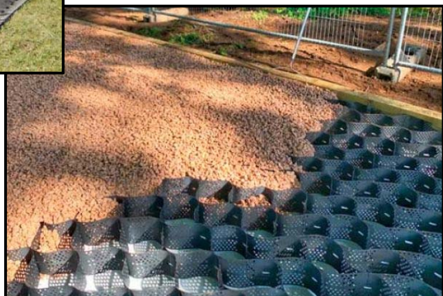
Right: Geoweb ground compaction mitigation (image www.greenfix.co.uk )
