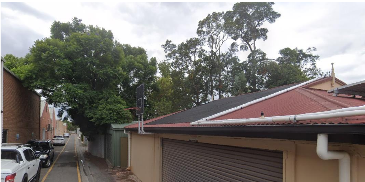
Figure 3 – View of the trees from rear laneway, facing north
