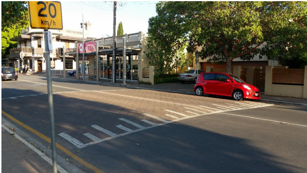
Figure 4.3: Example of Raised Table Treatment with On-street Parking and Access Maintained
