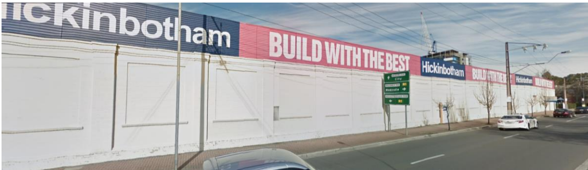
Photograph 1. View of northern façade of the building at 30 North Terrace
