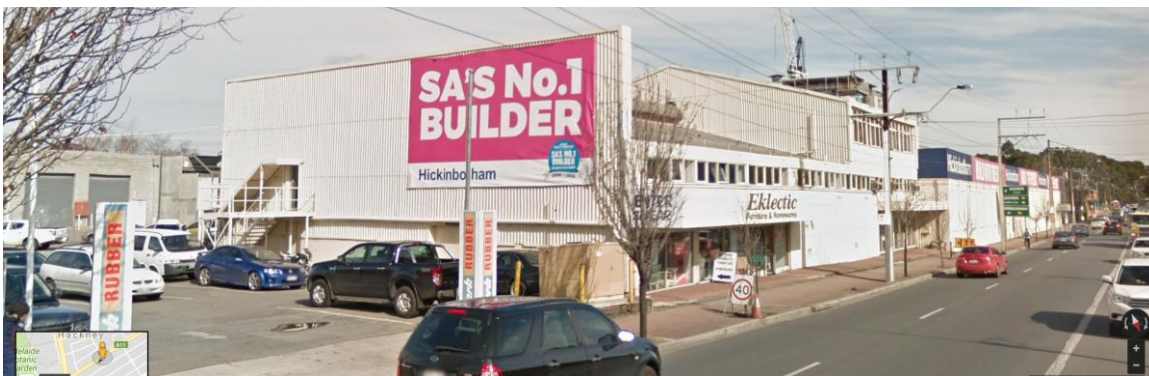
Photograph 2. View of eastern side of the building at 30 North Terrace
