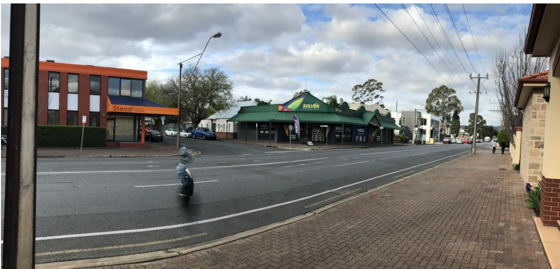
Photograph 1. View from Magill Road, approximately 80 metres west of the subject land
