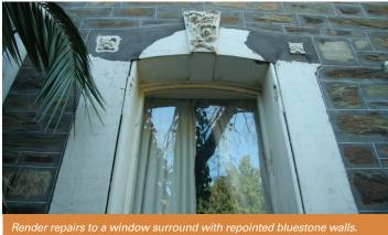
Older brickwork is usually pointed in a simple lime mortar. This is common on the sides and rears of houses, and less opulent or earlier houses. Like stone however, on more opulent buildings red oxide-coloured pointing was often used, with white or black line marking.
