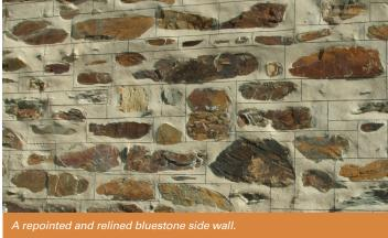
The mortar which binds stones or bricks together should always be weaker than the stone or brick so that it can fail first, not the other way around. An impervious bedding or pointing mortar (one made with Portland cement) can accelerate the deterioration of an older masonry wall. It is important that the tradesperson doing the repointing work knows how to work with lime.
